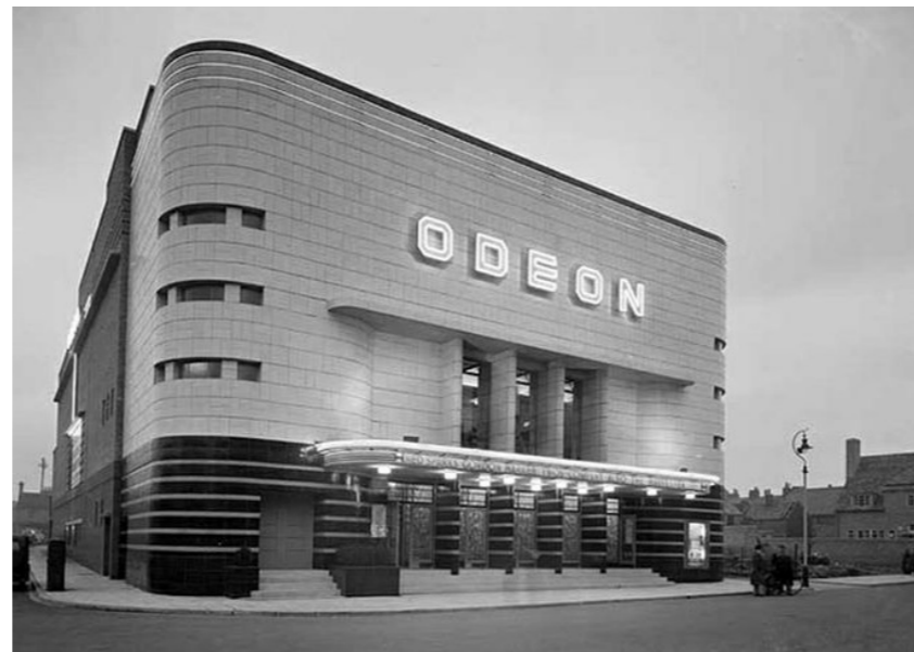
Example of free standing cinema - Odeon cinema, Loughborough
