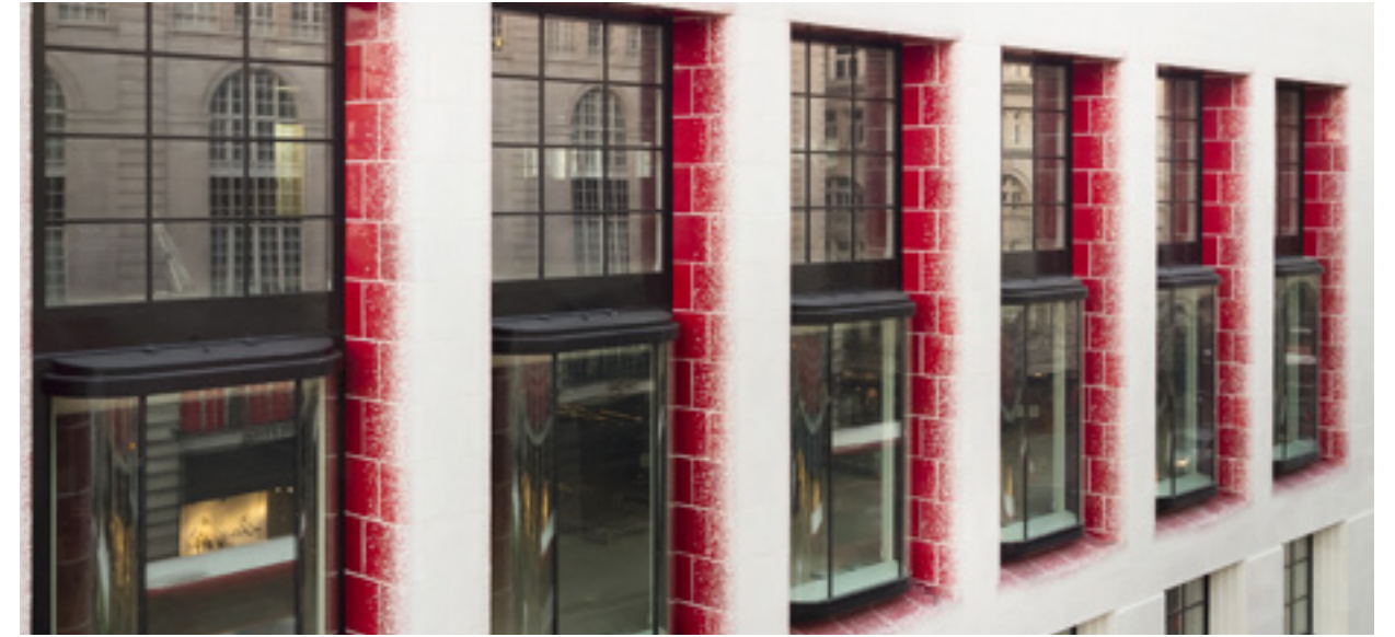
Example of tiled reveals to glazed openings - providing emphasis to reveal when viewed from an oblique angle
