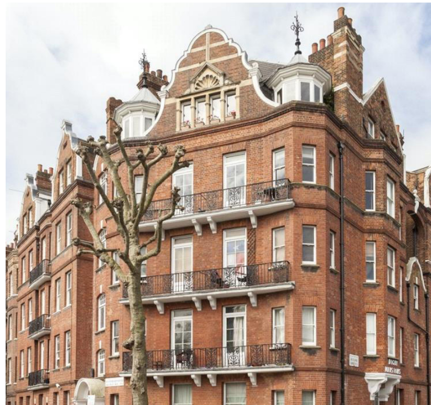
Digby Mansions (street facing facade)
