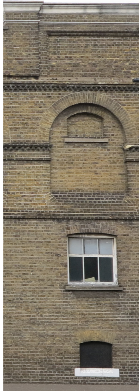
Existing photograph of openings facing the High Street
