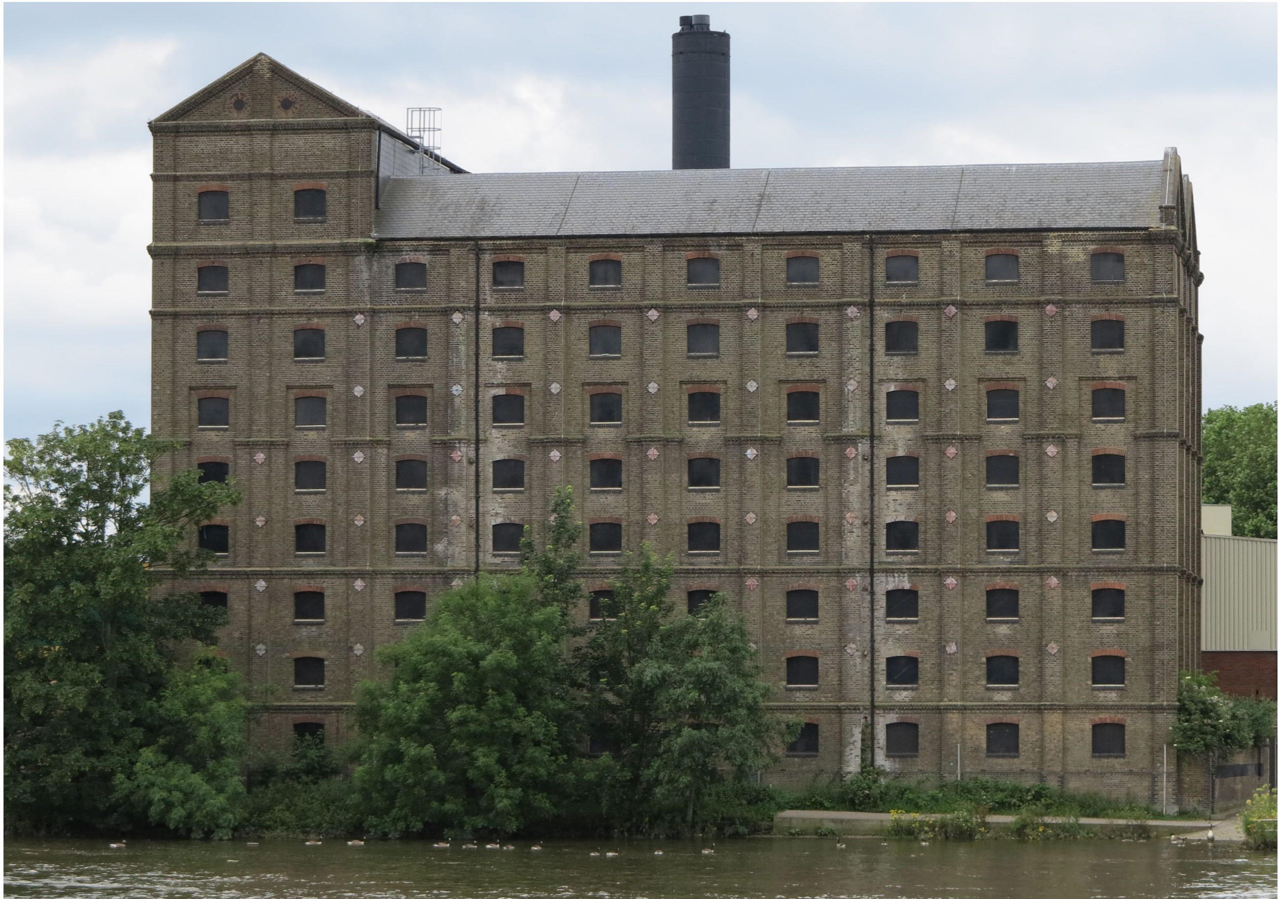
Photograph of existing Maltings building
