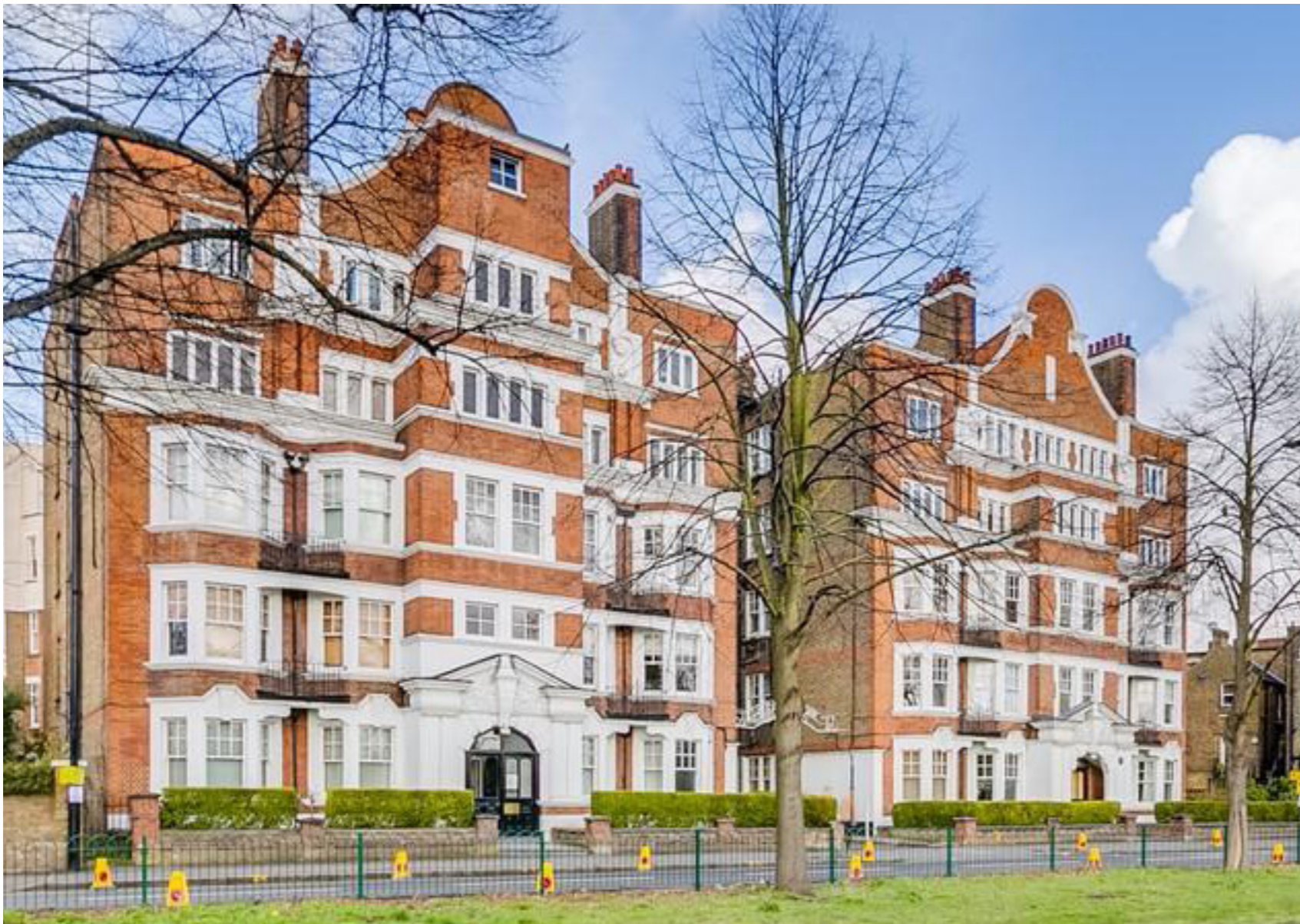
Exterior photograph of Arlington Park Mansions
