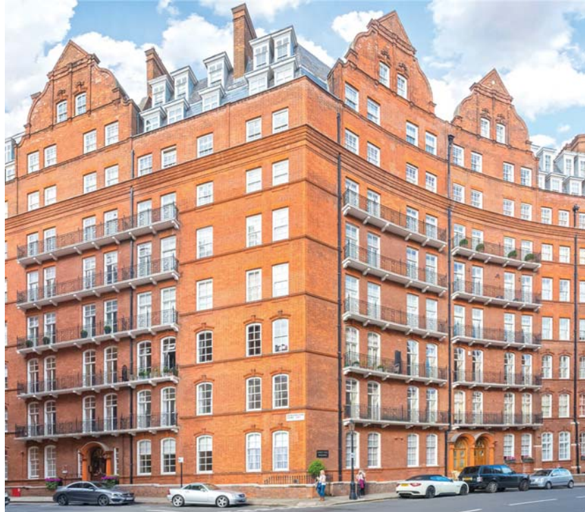
ALBERT HALL MANSIONS: DOUBLE MANSARD ROOF ERODES TOP OF BUILDING
