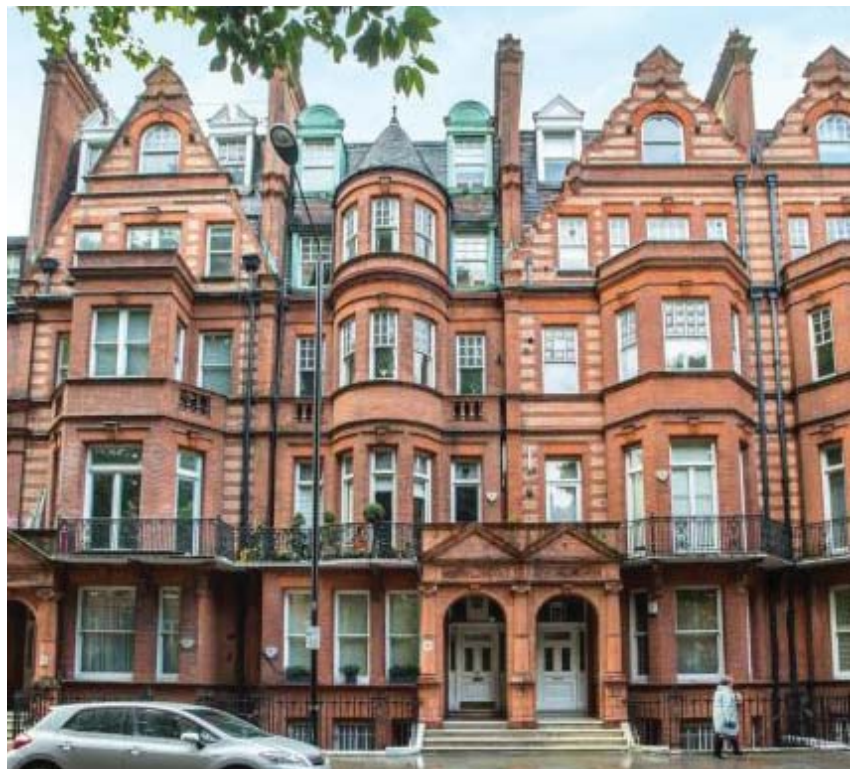
SLOANE GARDENS: DOUBLE MANSARD, DORMER WINDOWS & VARIED GABLES
