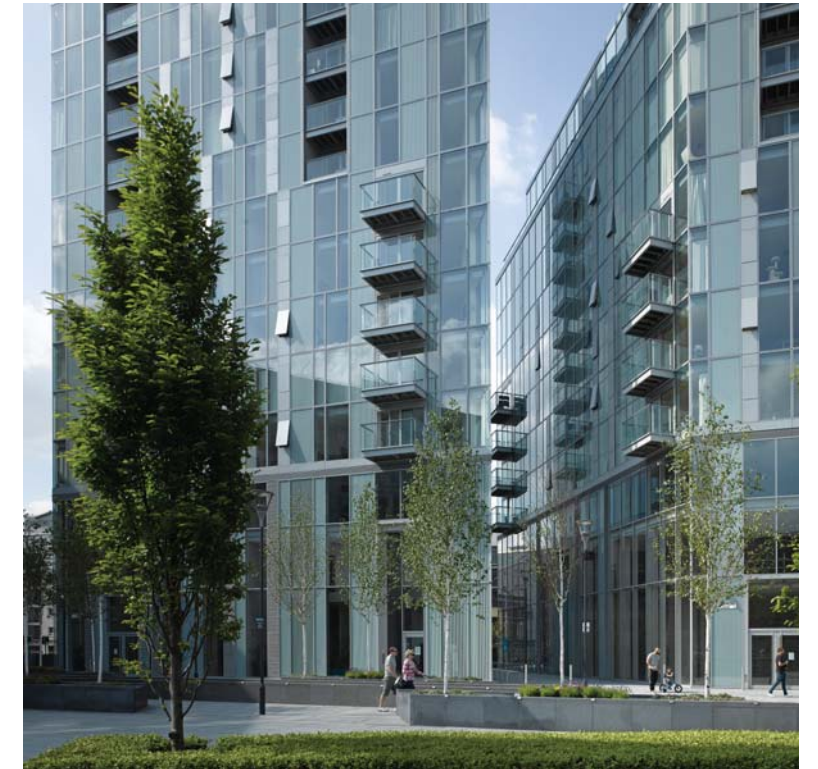
Creekside West - Photograph
