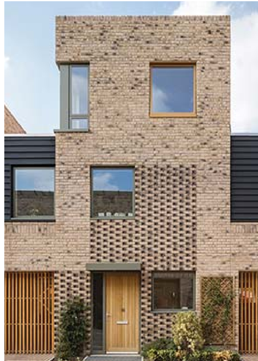
Example of timbers secondary elements only
