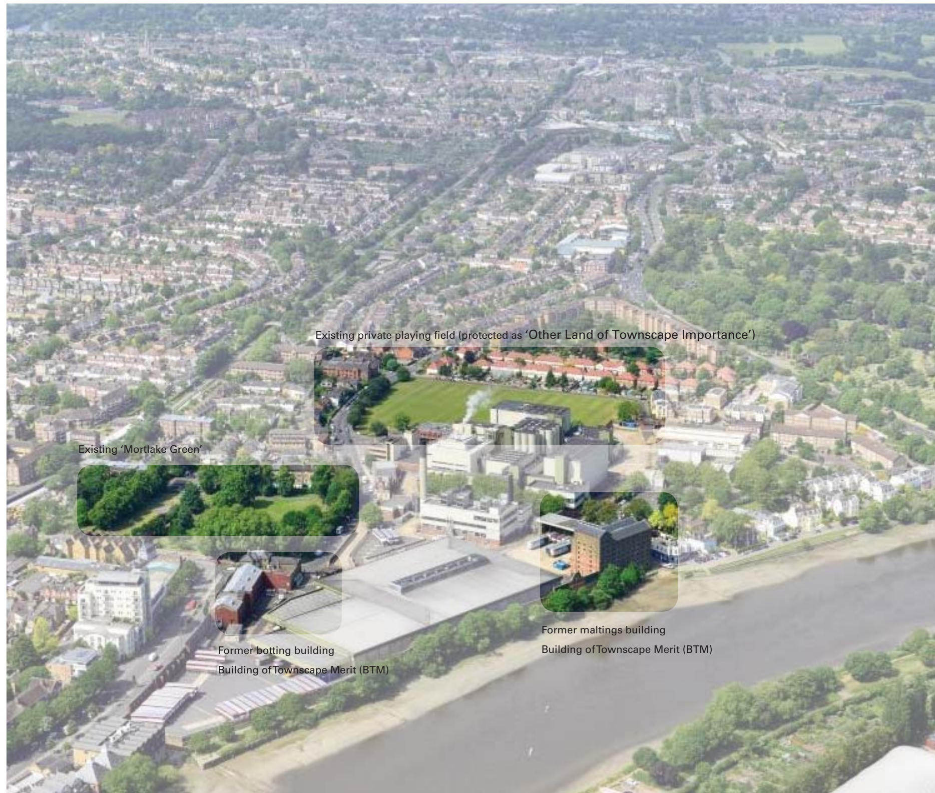
Bird's eye view of existing site - key features of existing site and context highlighted
