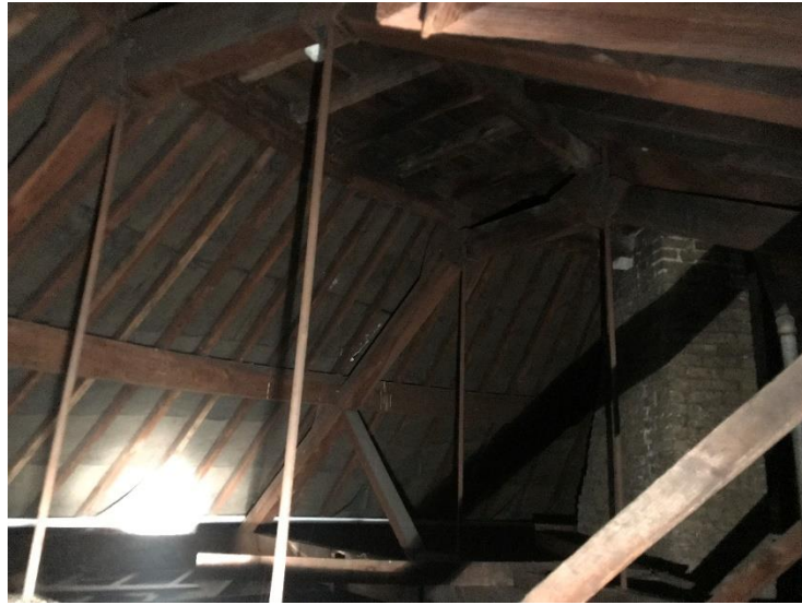
Plate 9 – South-western loft space of building B10.
