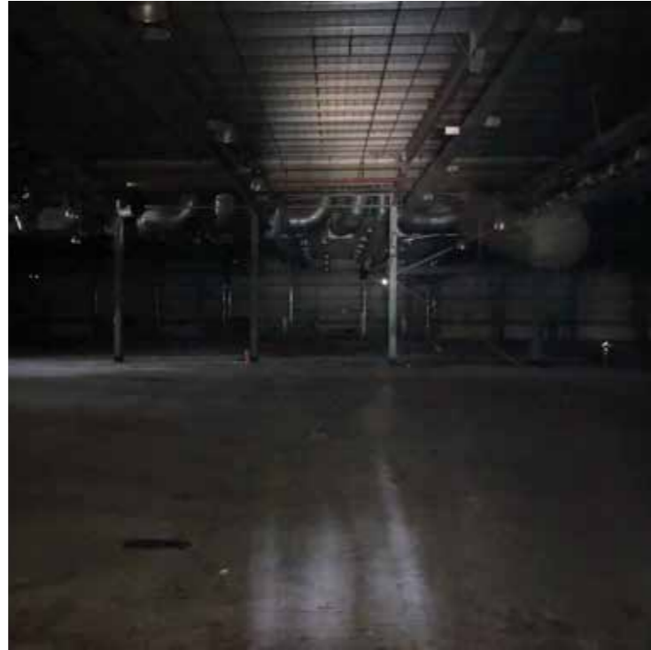
Interior of eastern area bottling warehouse with stripout completed
