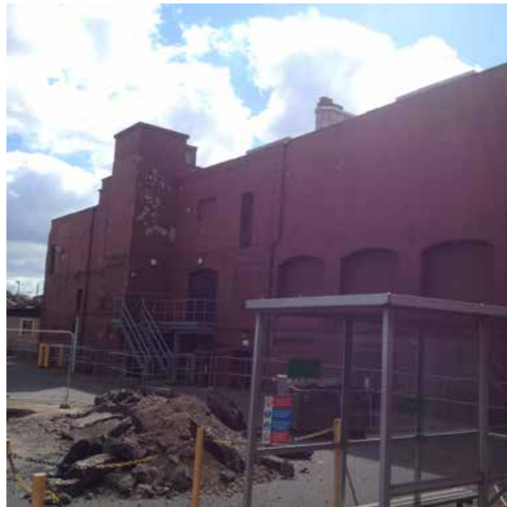
The (former) Bottling Hall
