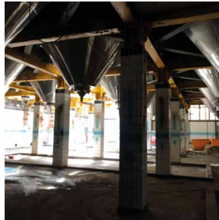
Further tanks in brewhouse awaiting removal
