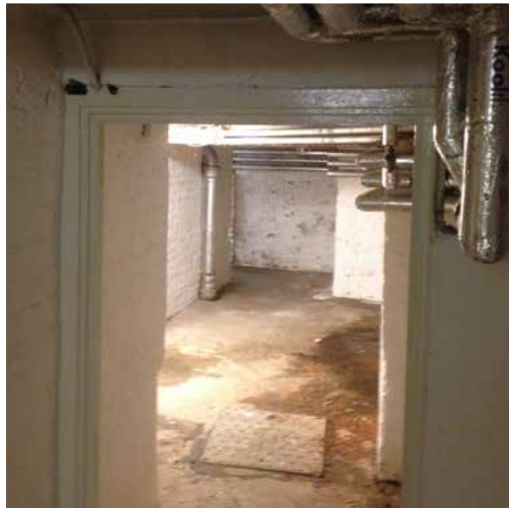
The (former) Hotel cellar used as the staff canteen
