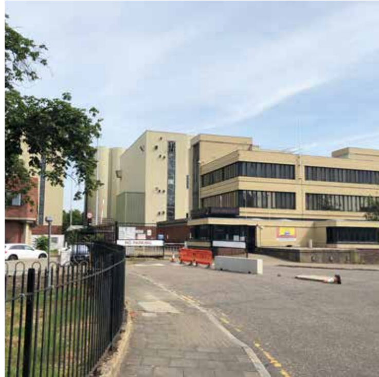
Site entrance at western area
