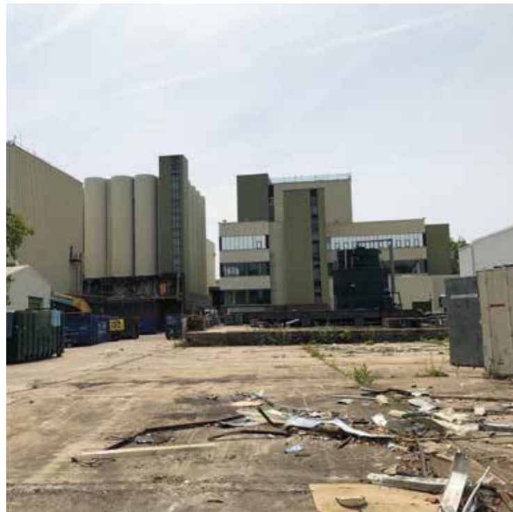
Former base for removed effluent tank
