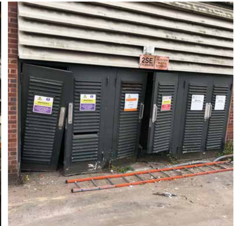
Emptied chemical storage sheds at brewhouse
