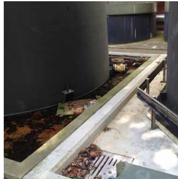
Condition of tank sumps
