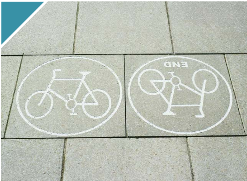
Artificial Stone Flag Paving
