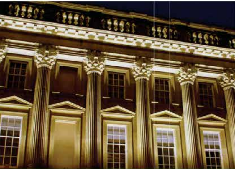
External lighting for historic buildings
