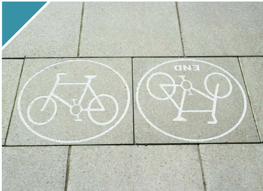
Artificial Stone Flag Paving
