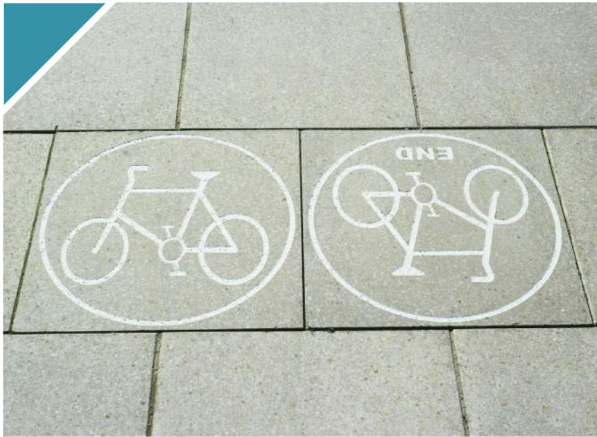
Artificial Stone Flag Paving
