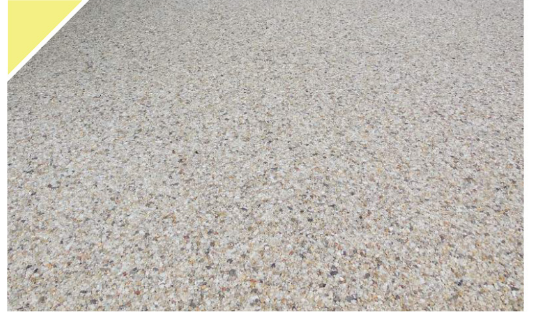
Resin Bound Aggregate Paving
