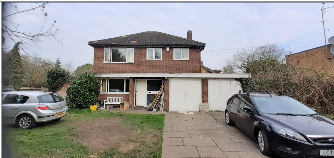
Photo 2: Looking west at the east elevation and entrance to the site from St. James's Road.
