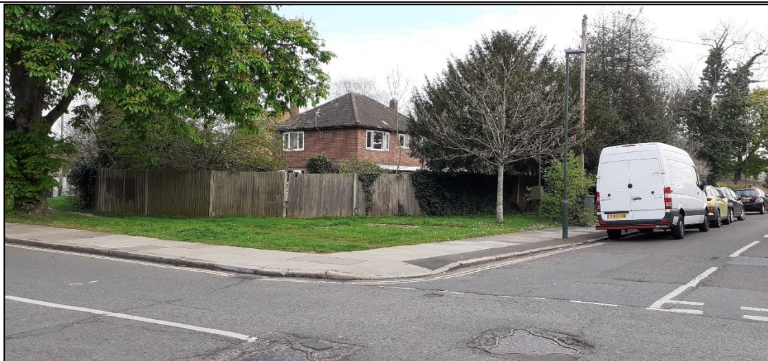
Photo 1: B1 - Looking north-west at the south-east elevation of the site from the pavement opposite on Windmill Road.
