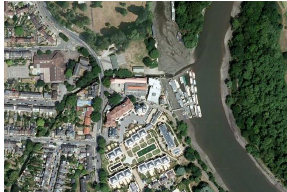
Figure 1: An aerial view of the site which illustrates its proximity to the Thames and the World Heritage Site buffer zone.
