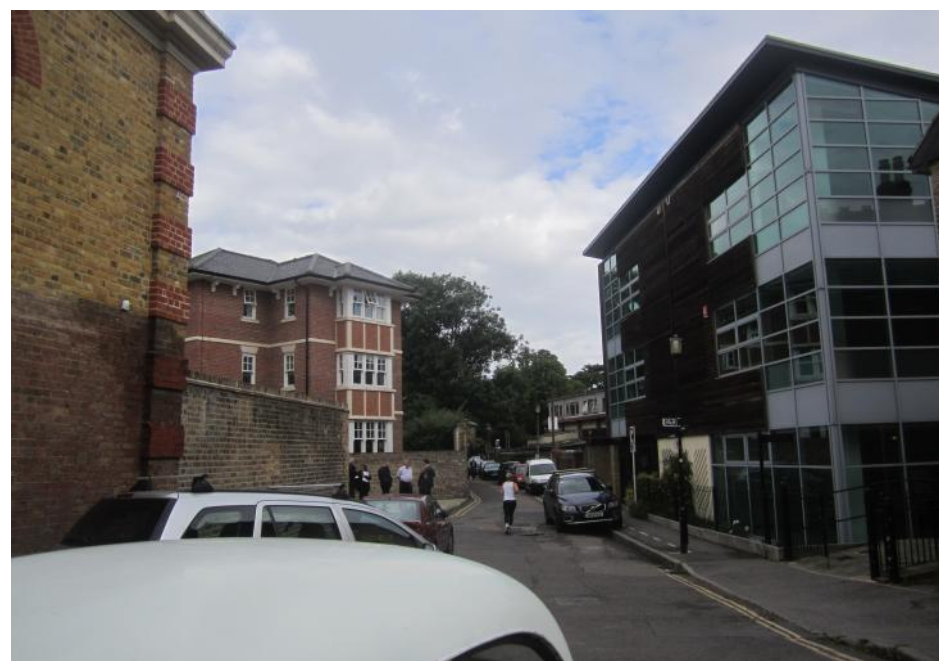
Figure 15: A view of the proximity of the former stable block (seen to the left of this photograph) to the existing built environment along Railshead Road.
