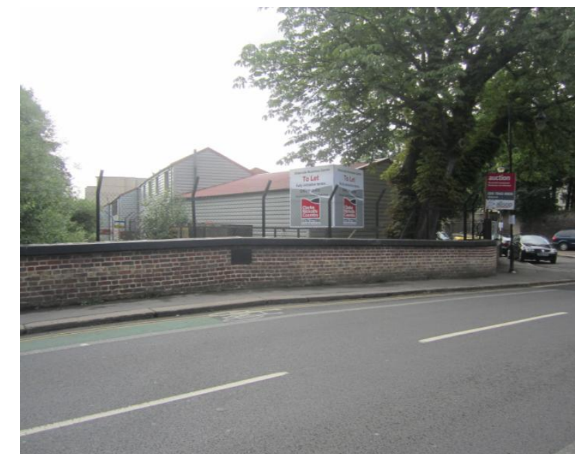
Figure 16: The view towards the site as taken from Railshead Bridge. The views of the rear of the existing warehouse buildings present a negative frontage within the Conservation Area.
