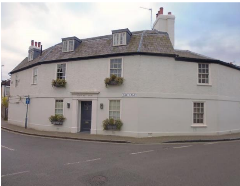
Plate 17: Grade II Listed Devoncroft House.
