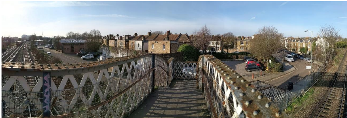
Site from Rail Foot Bridge (looking north)
