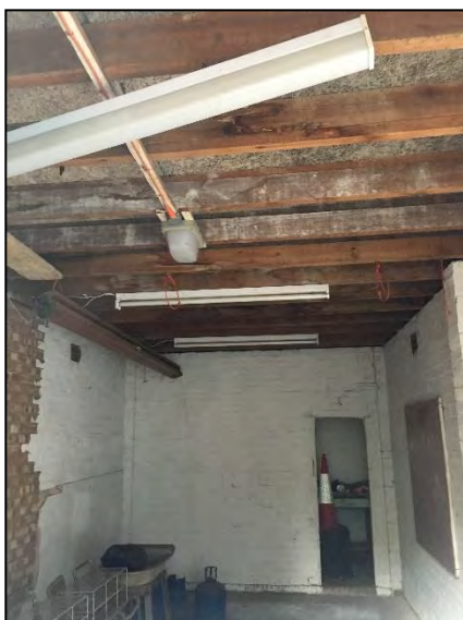
Photograph 18: Interior of building 2
