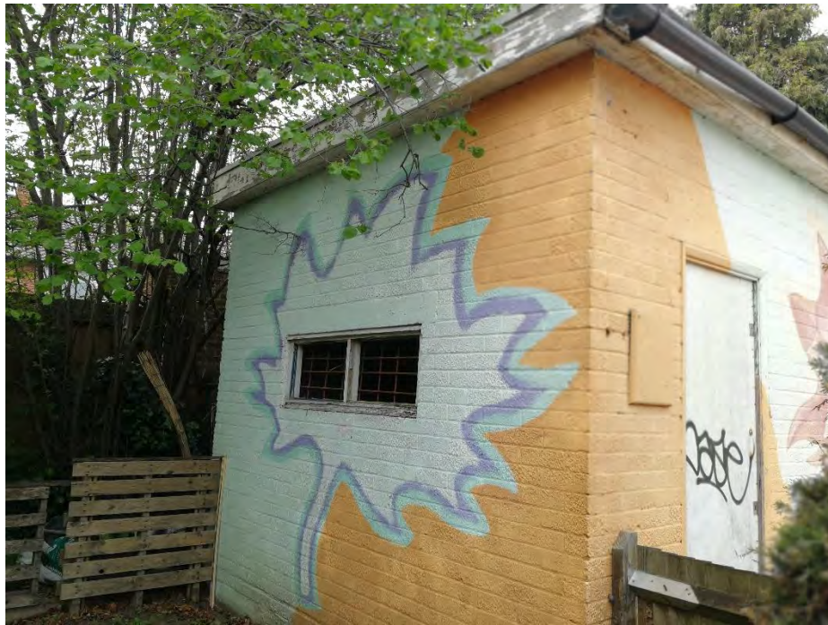
Photograph 4: View of Building 2 with the open window at the western border of the Application Site.
