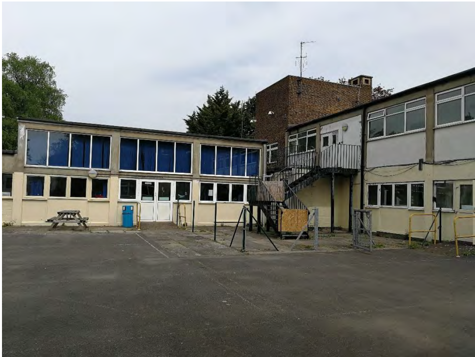
Photograph 3: View of hardstanding and western elevation of Building 1 at the northern end of the Application Site.
