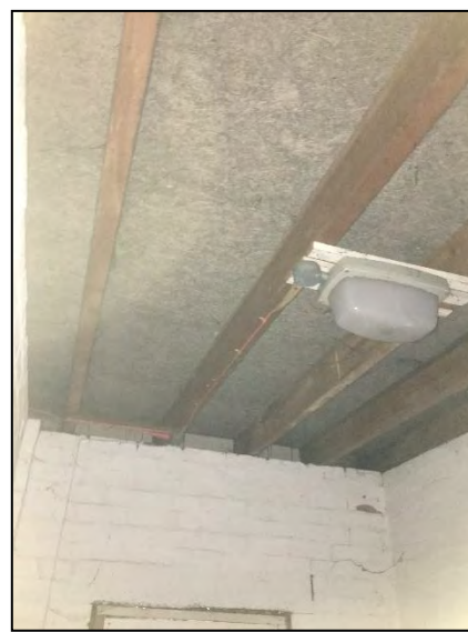
Photograph 19: Interior of building 2
