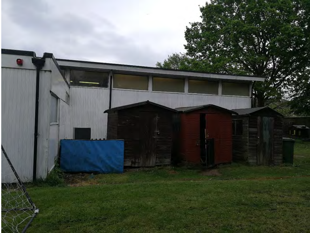
Photograph 6: View of Building 6, the large nursery building in the southern end of the Application Site accompanied by the three small wooden sheds (Buildings 7, 8 and 9).
