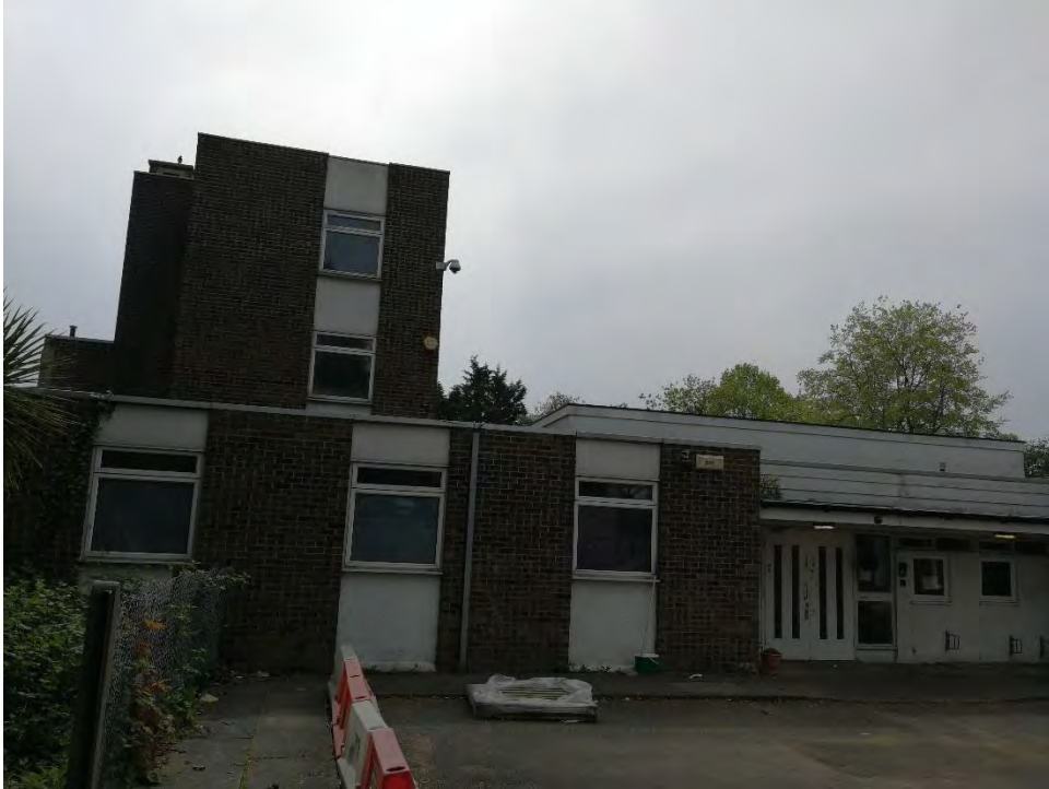
Photograph 2: View of hardstanding and northern elevation of Building 1 at the northern end of the Application Site.
