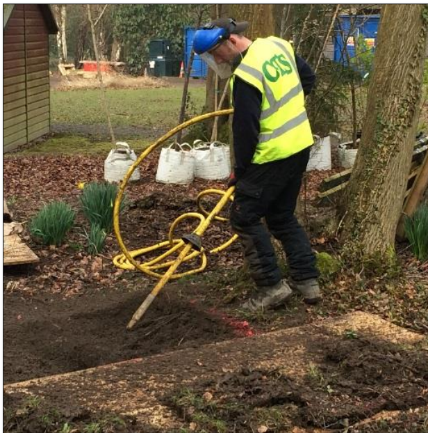
Fig. 2 Use compressed air to remove soil from roots
