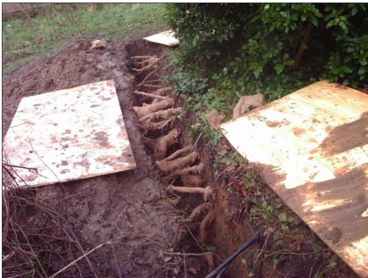
Fig. 4 Roots wrapped for identification and assessment by the appointed arboricultural consultant
