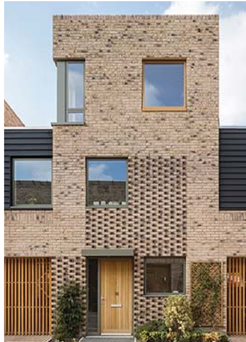
Example of timbers secondary elements only
