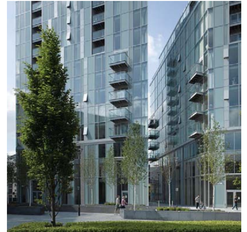
Creekside West - Photograph
