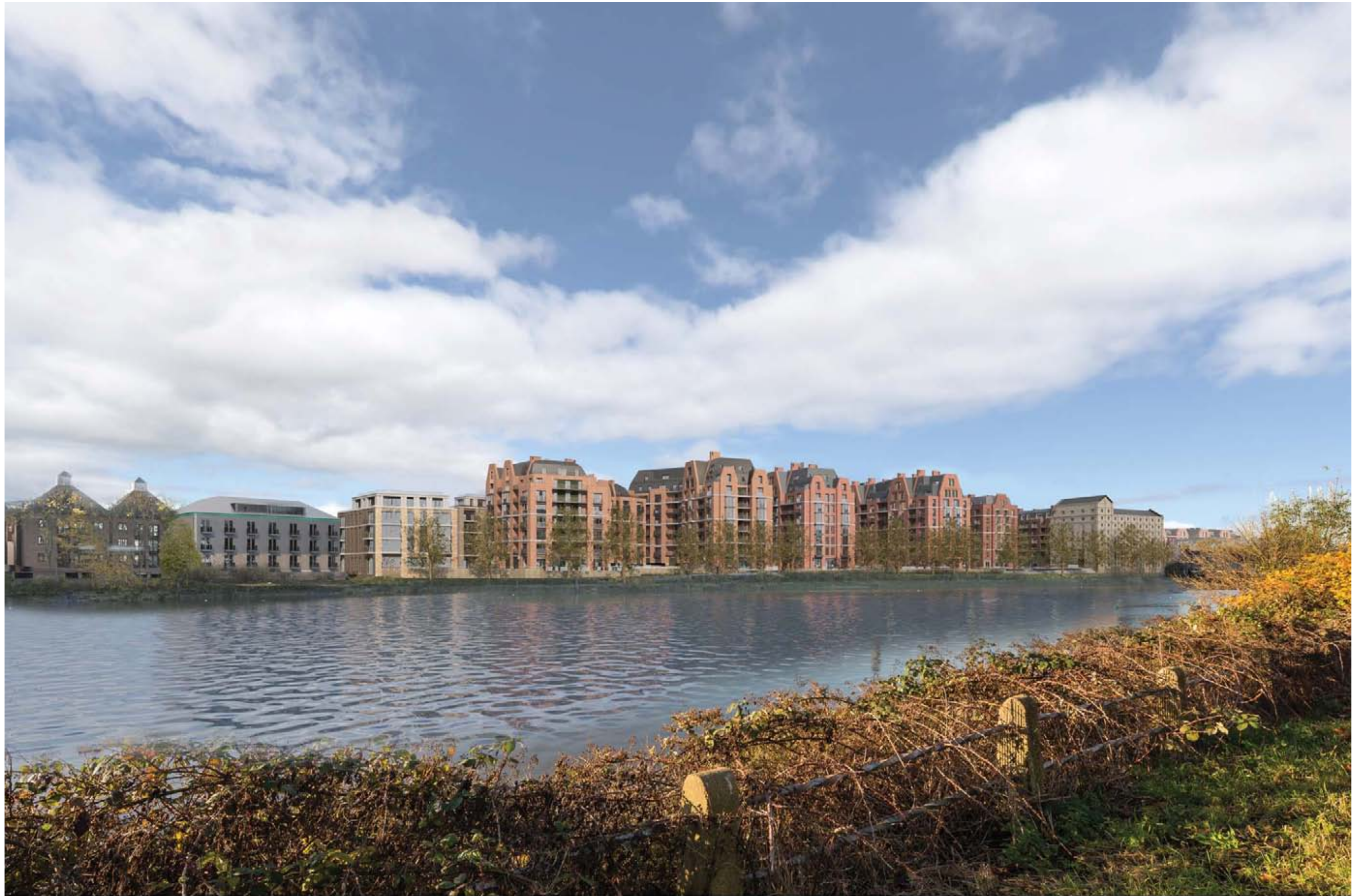
VIEW FROM NORTH EAST
