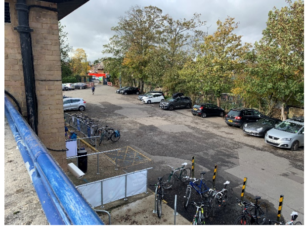
View of main building and car park.
