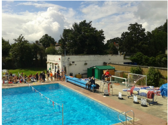
View of the pool and pump room/ maintenance Building, looking south-west.
