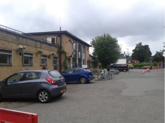
View of the main building and car park, looking west.
