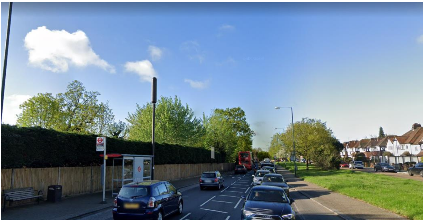
Image 1: Existing 2G/3G/4G site
