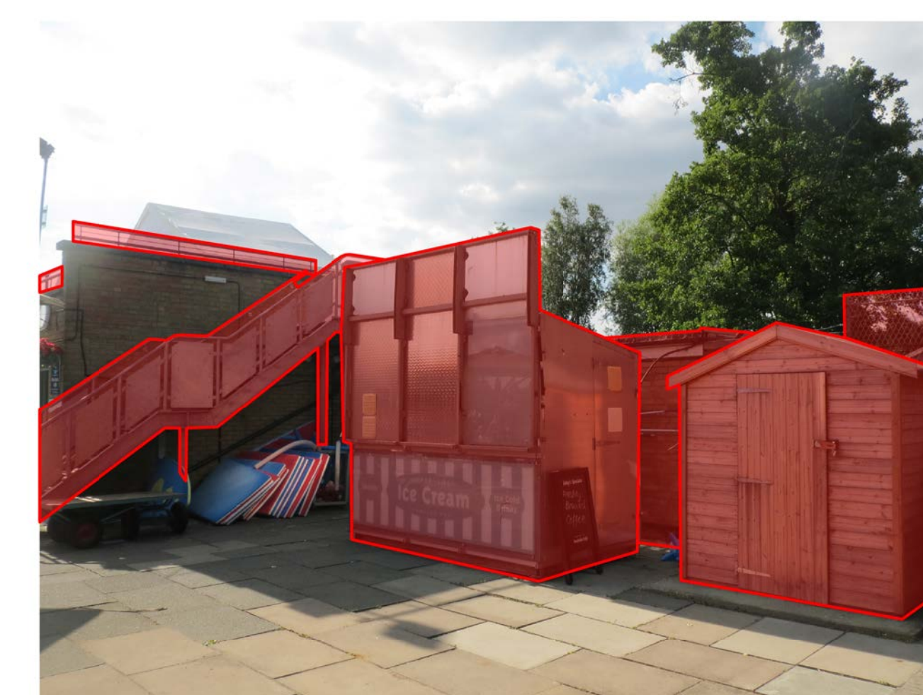
East end of existing building
