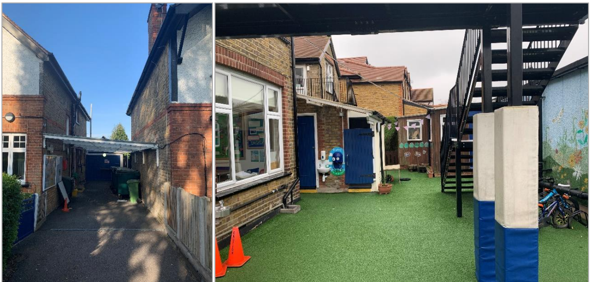
Figure 4: Side Access and External Staircase and WC
