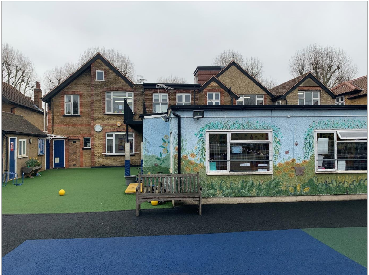
Figure 5: Existing Kindergarten Building
