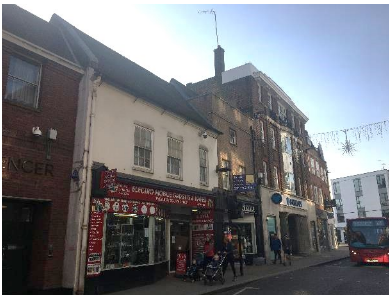
Plate 5: Front elevation from street-level.
