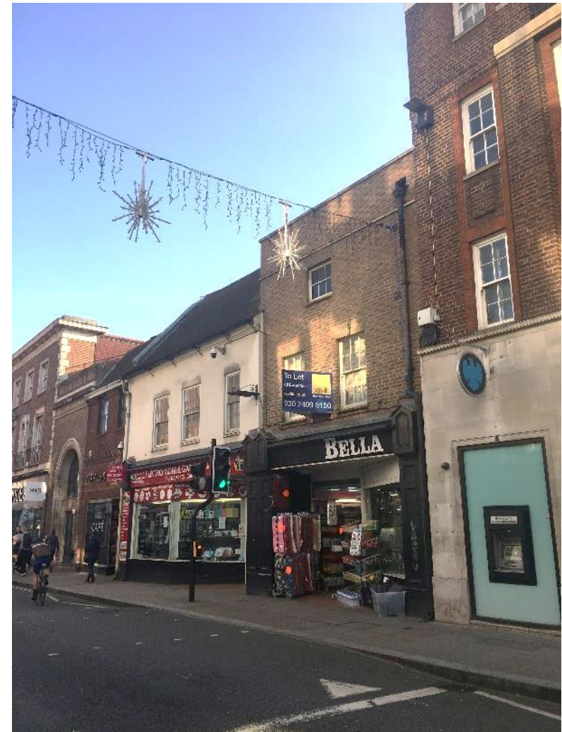
Plate 4: Front elevation from street-level.
