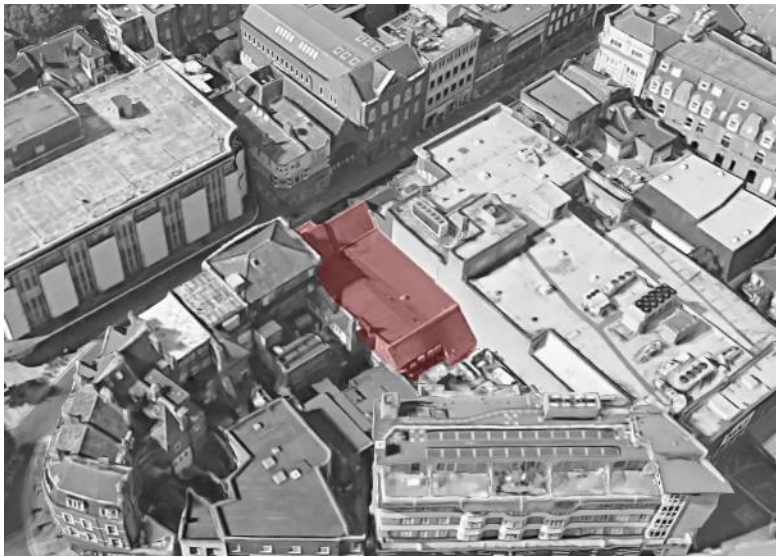
Plate 3: Aerial view of the rear elevation and roof.
