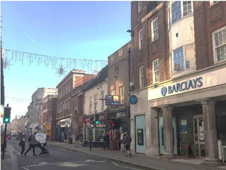
Plate 15: Existing view from the west.
