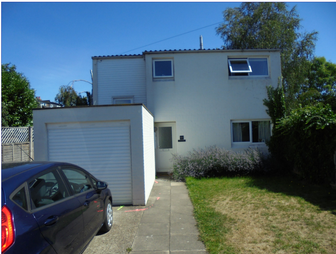
Plate 2: Northeast facing view of the front elevation of 32 Cross Street
