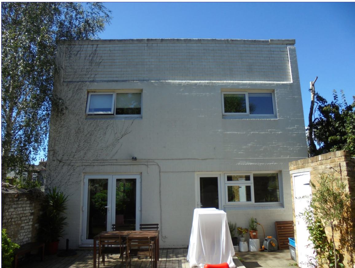
Plate 4: Southwest facing view of the rear elevation of 32 Cross Street
