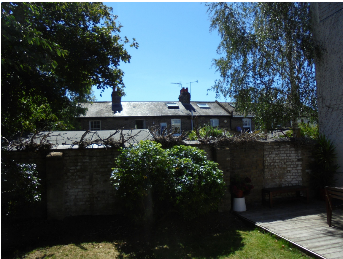
Plate 6: Southeast facing view of boundary wall to the rear of 32 Cross Street on the southeast side of the Site
