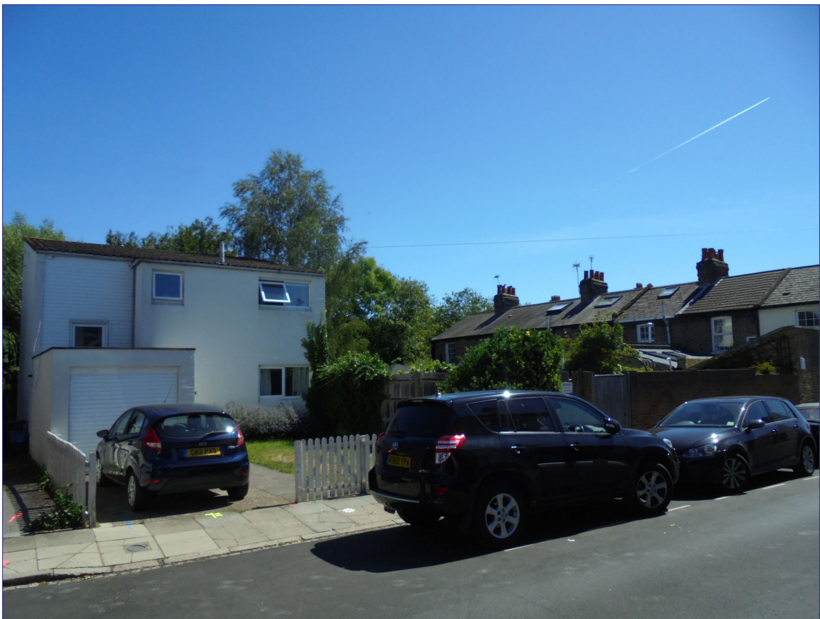
Plate 8: East facing view towards the Site and the rear of Numbers 50 to 56 Railway Side
