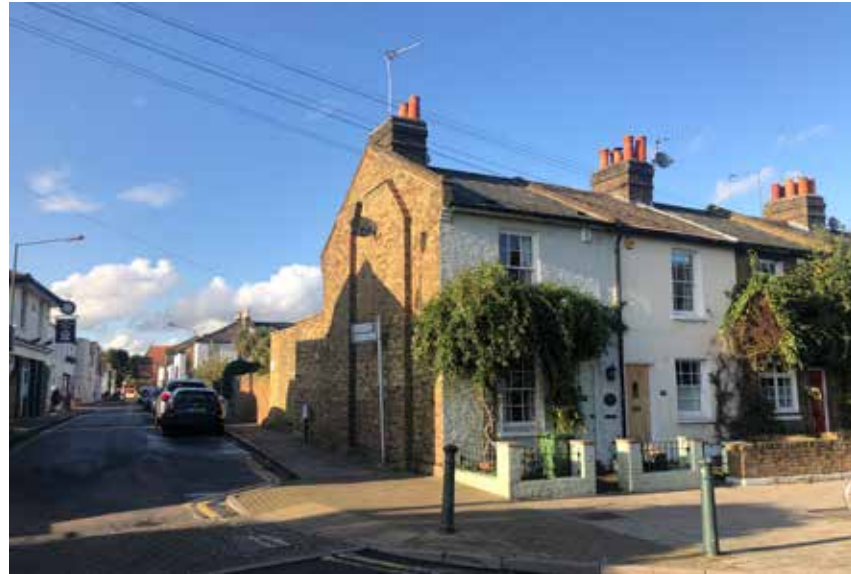
Front wall of the 50-56 Railway Side. Northwest view
