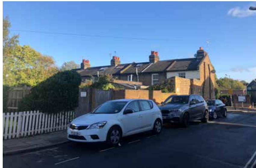
Flank and back wall of the 50-56 Railway Side. Southeast view
