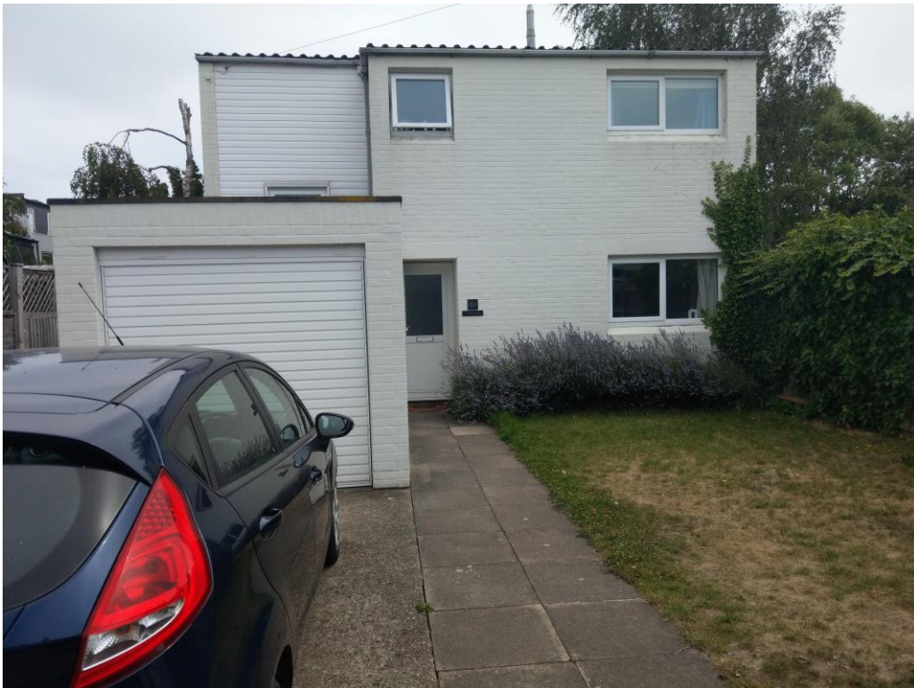
Photo A3.1: Front of caretaker's cottage (south west facing)
