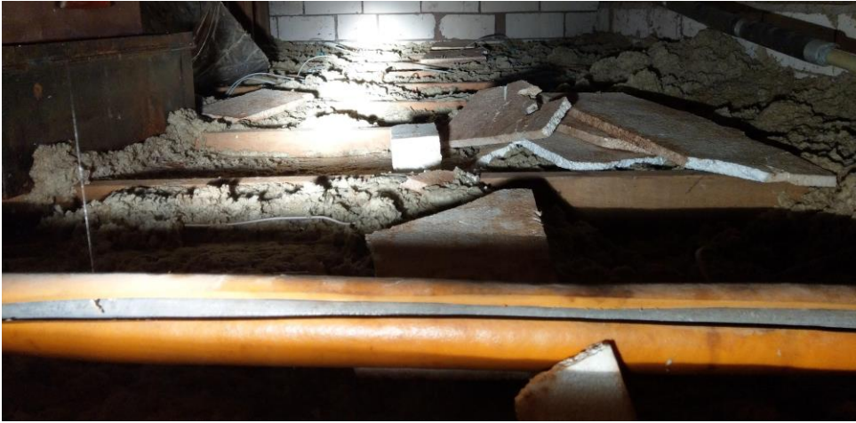
Photo A3.4: Internal roof void
