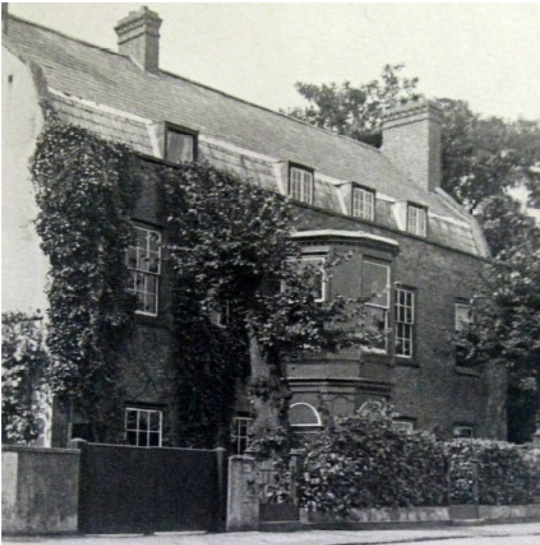
View of the frontage of Leyden House in 1944
