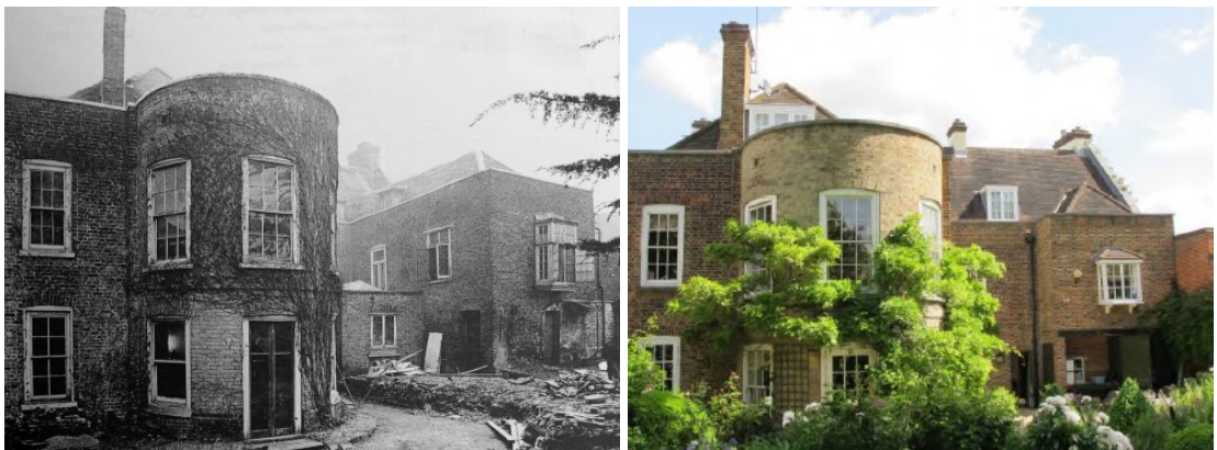
Further view of rear showing east wing before removal (1961) and simialr view as of 2019
