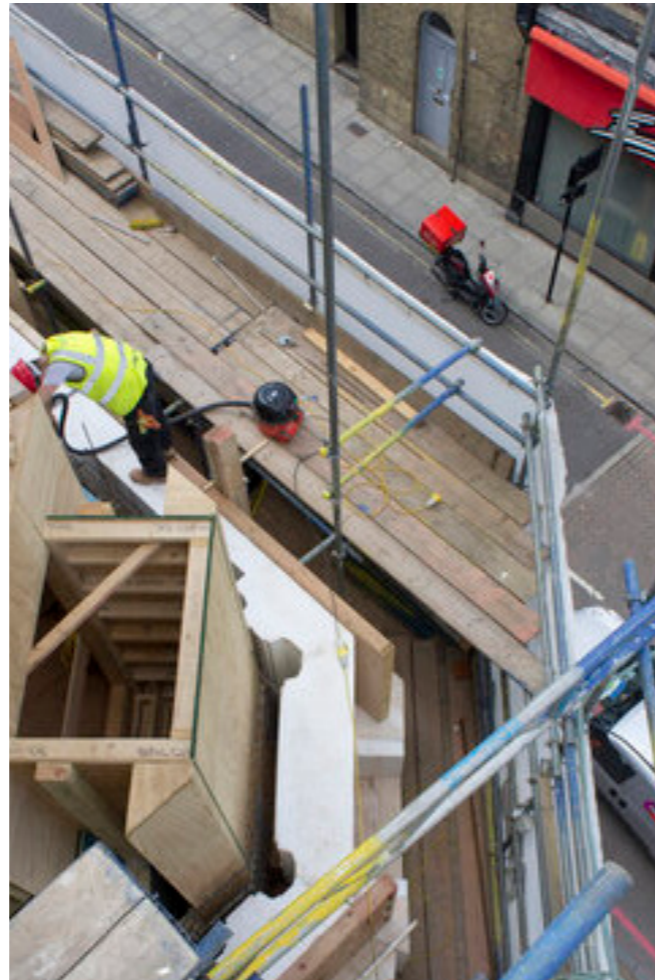
Framework installed on-site
