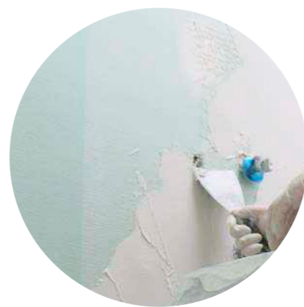
New Micro-cement Coating
