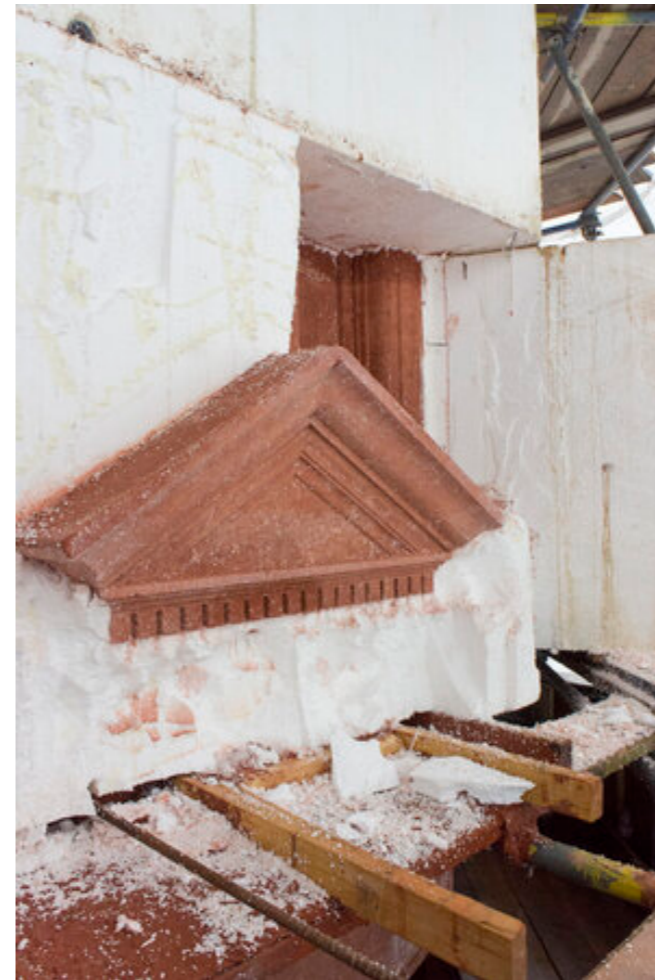
Cutting framework away to reveal concrete:
