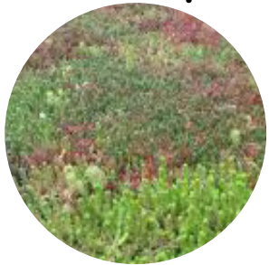
New green roof covering with pebble border
