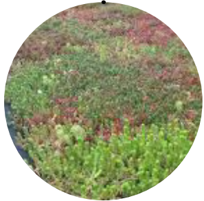
New green roof covering with pebble border
