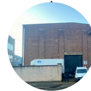
Existing brickwork to be cleaned up and enhanced
