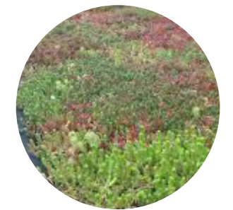
New green roof covering with pebble border
