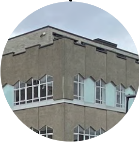
Existing concrete pebble dash to be retained and enhanced
