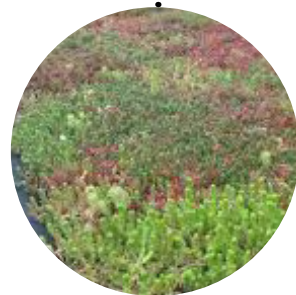
New green roof covering with pebble border
