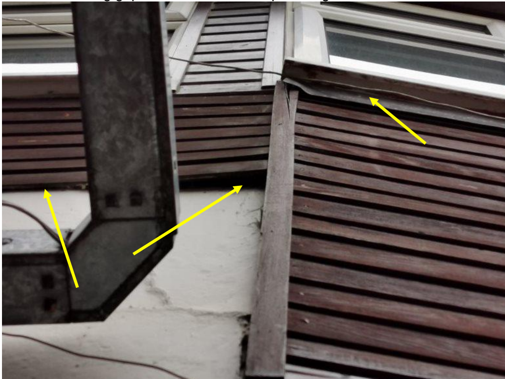
Plate 2: showing gaps under the wooden panelling
