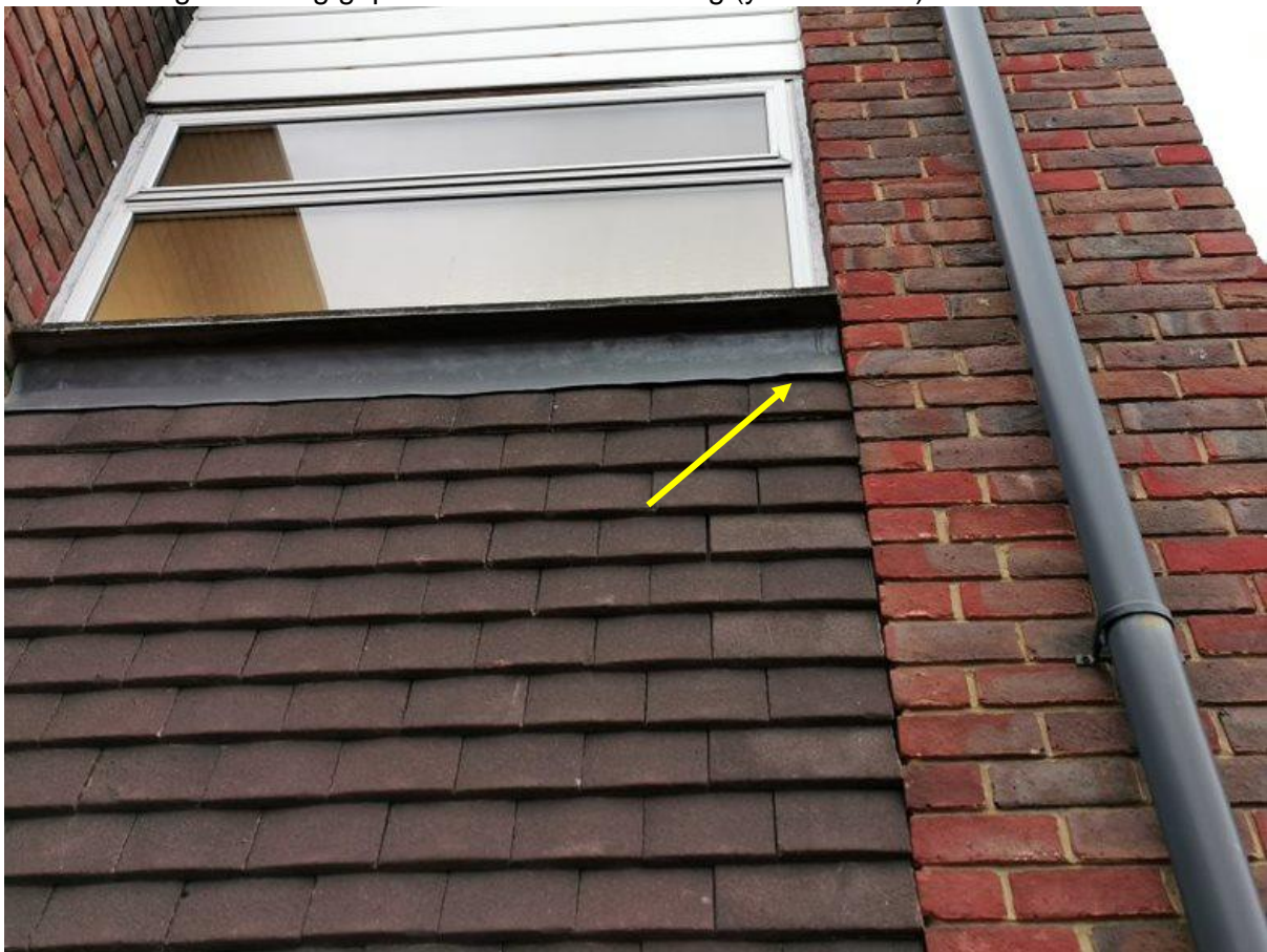
Plate 6: Image showing gaps under the lead flashing (yellow arrow).
