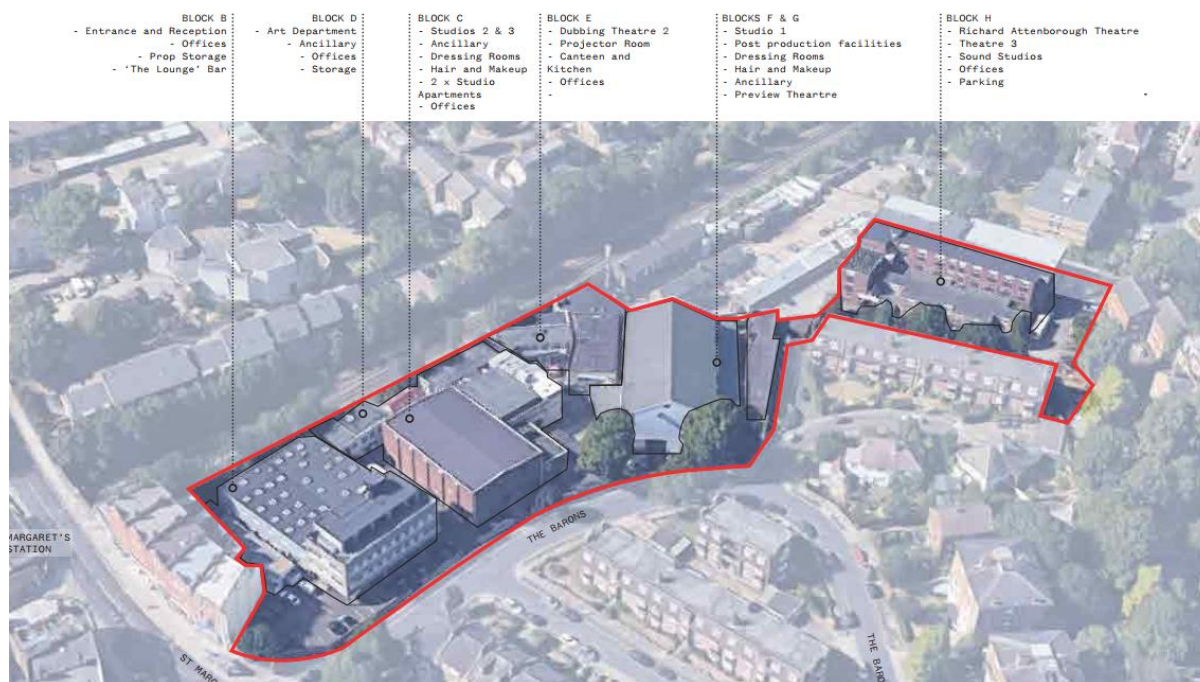
Figure 3: An aerial photograph of the current structures at Twickenham Film Studios (as shown by the red outline) taken from the pre-application Document.
