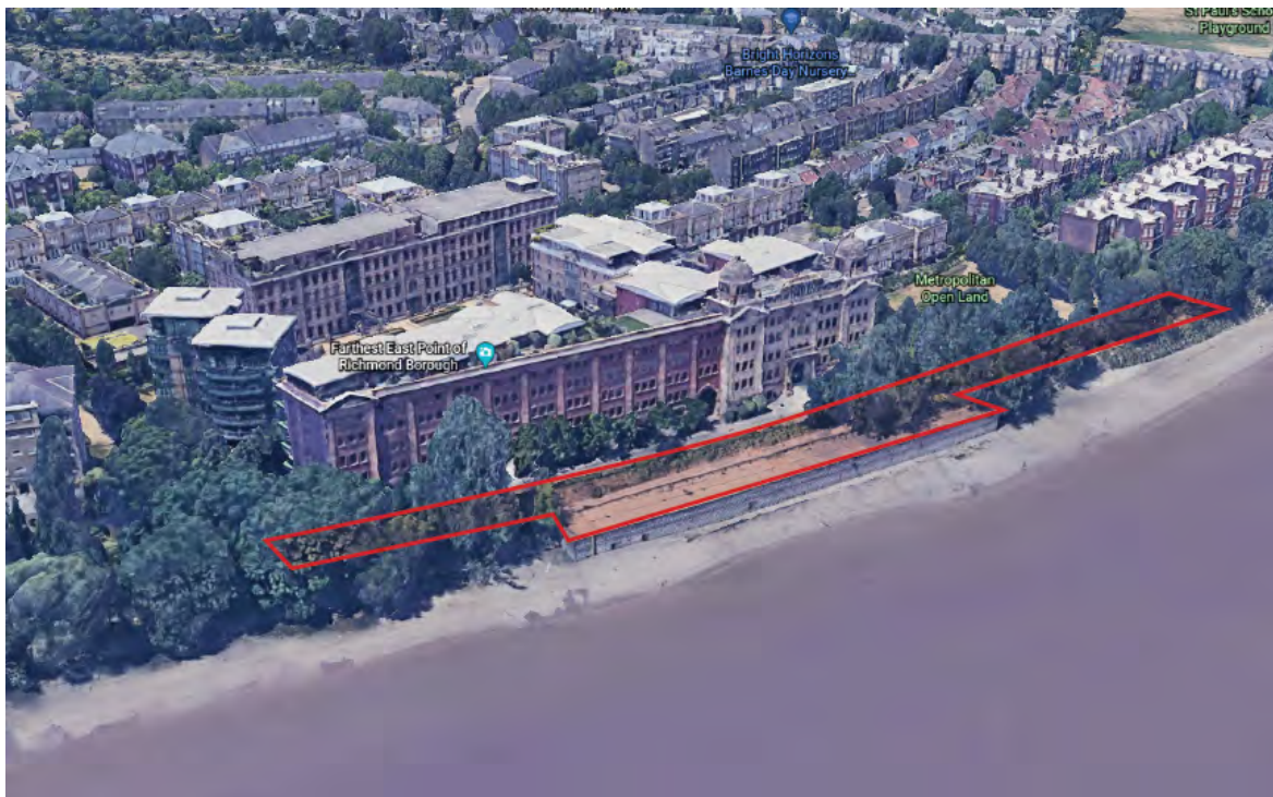
Photograph 1: Aerial view of application site looking west
