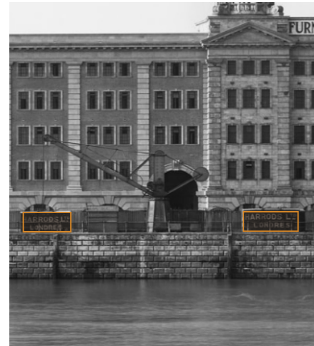
02 detail showing crates on the jetty, 1921
