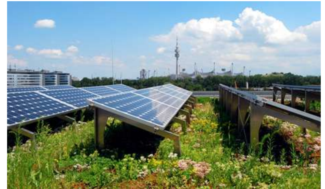
02 PV panels to roof
