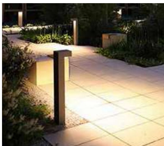
03 low level bollard lighting
