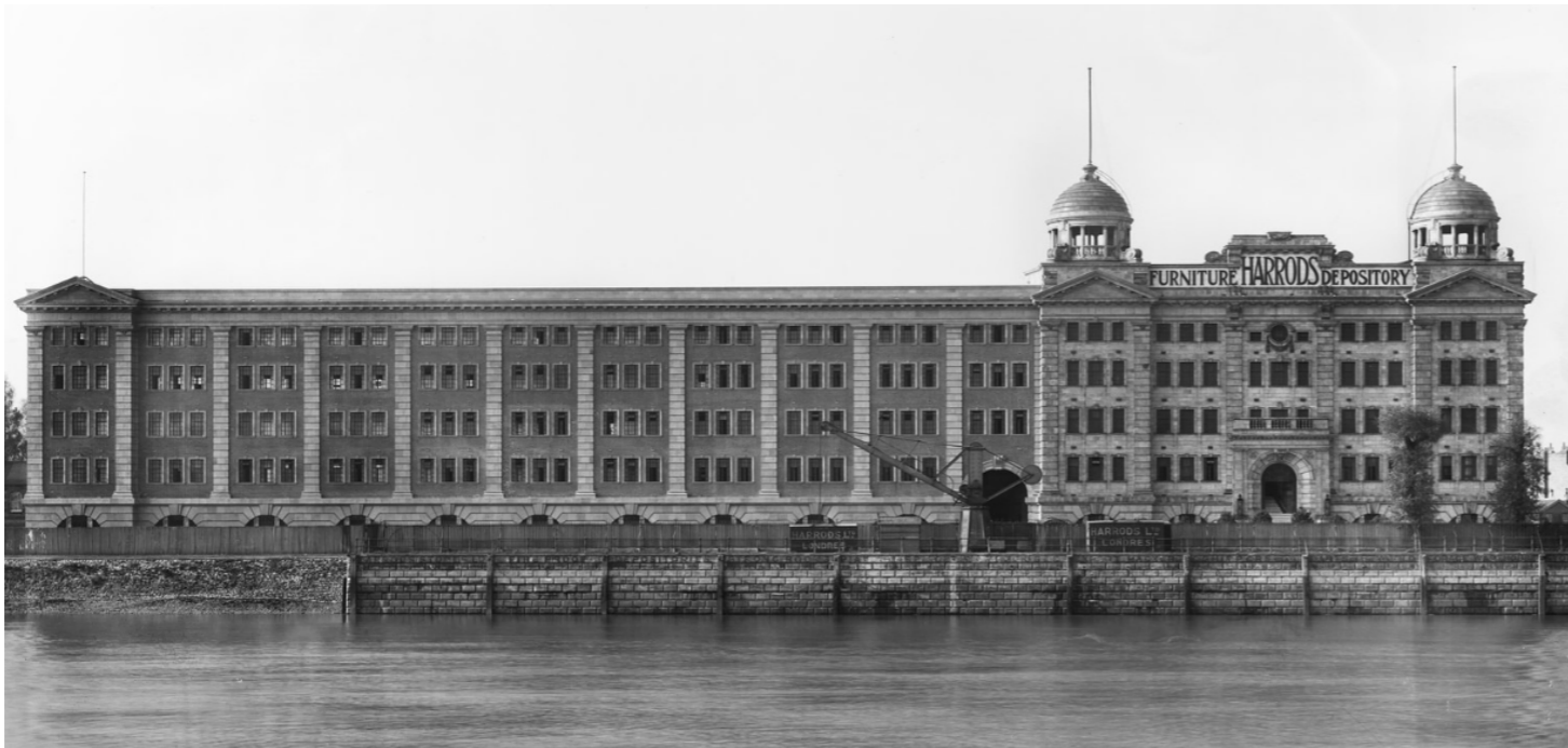
01 Historic image from Hammersmith looking west across Thames, 1921
