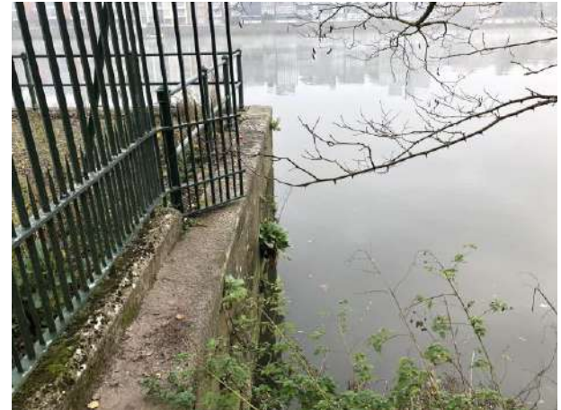
End of wharf where foliage can be seen in the wharf wall.
