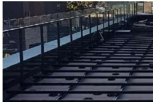
Typical deck support subframe
