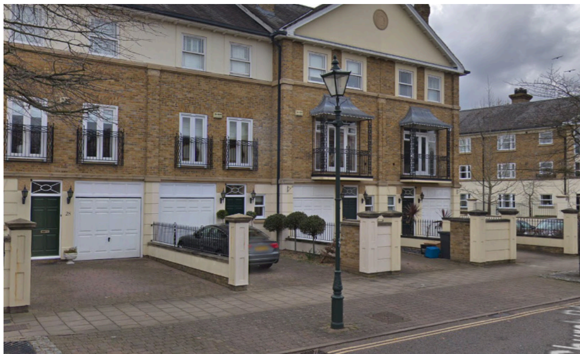
Current Street Lighting Provisions (Trinity Church Road)
