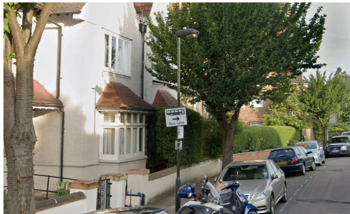
Current Street Lighting Provisions (Clavering Avenue)
