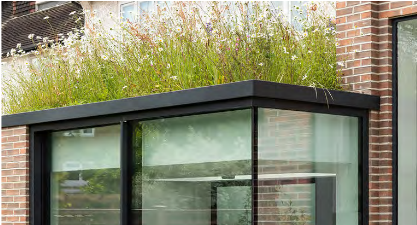
Semi-intensive green roof planted with a variety of native and ornamental perennials and grasses
