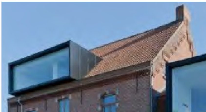
Zinc cladding on roof dormer
