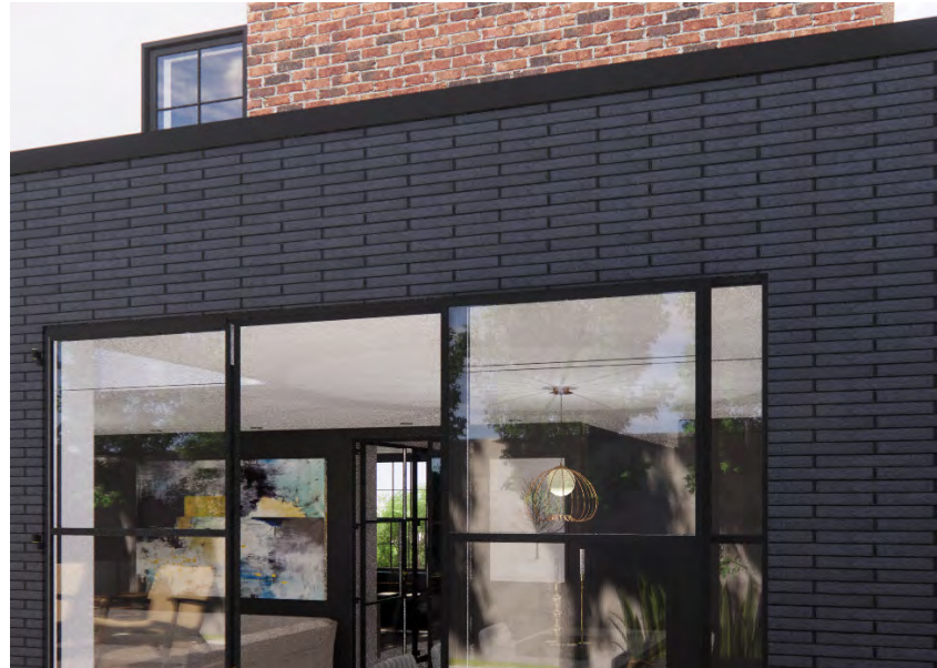
Black bricks and industrial style doors / crittal doors
