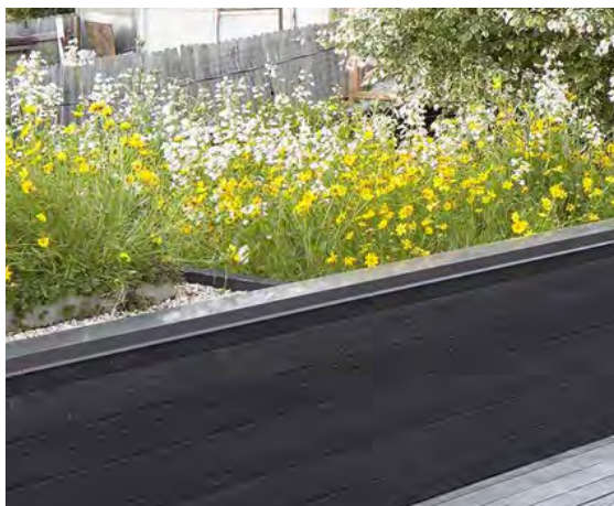
Semi-intensive green roof
