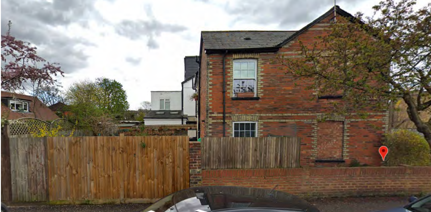
Wooden fence to be replaced by a brick wall of matching height. Original bricks to be re used as much as possible.
