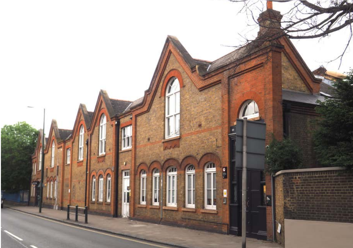
General view from Mortlake High Street
