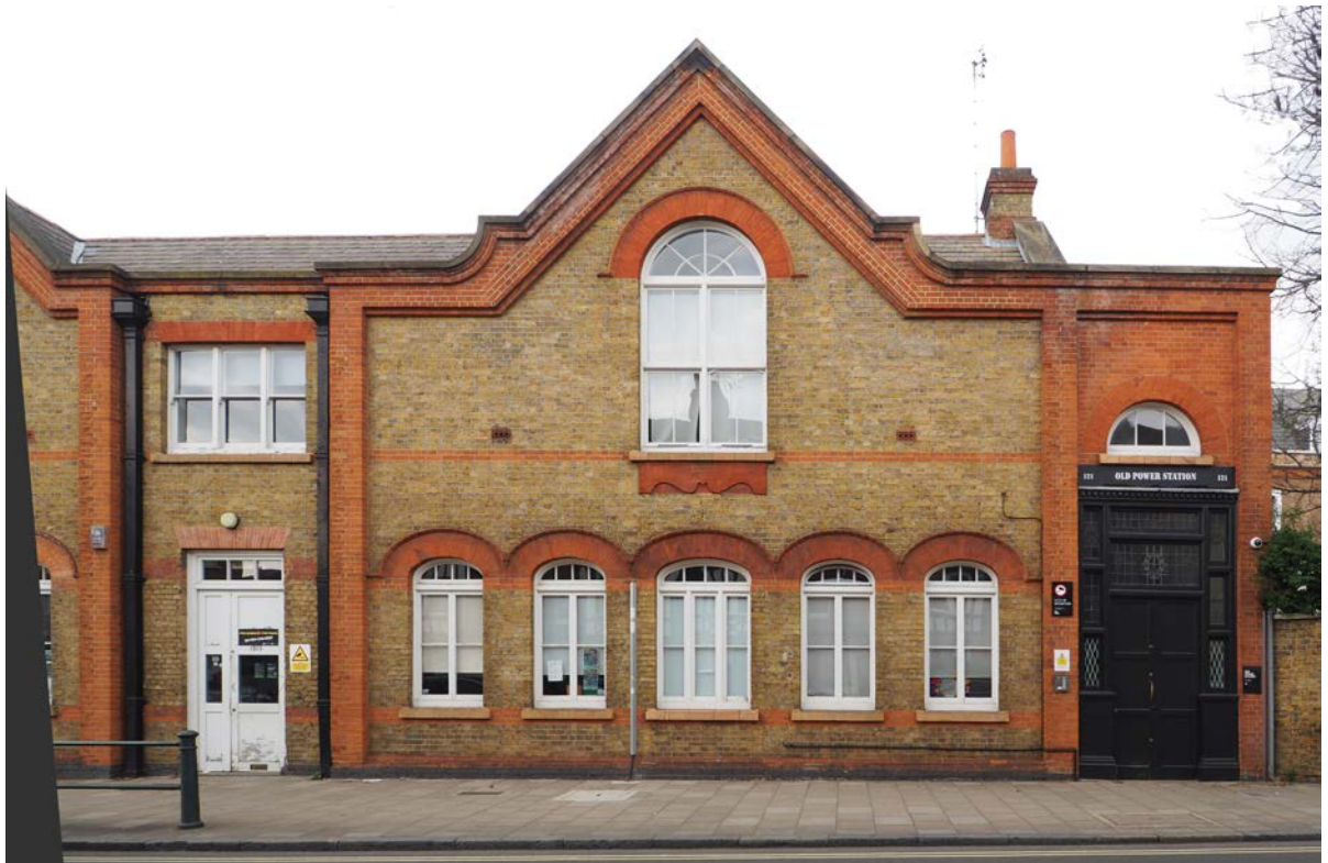
Left to right image 3, South Elevation of The Old Power Station
