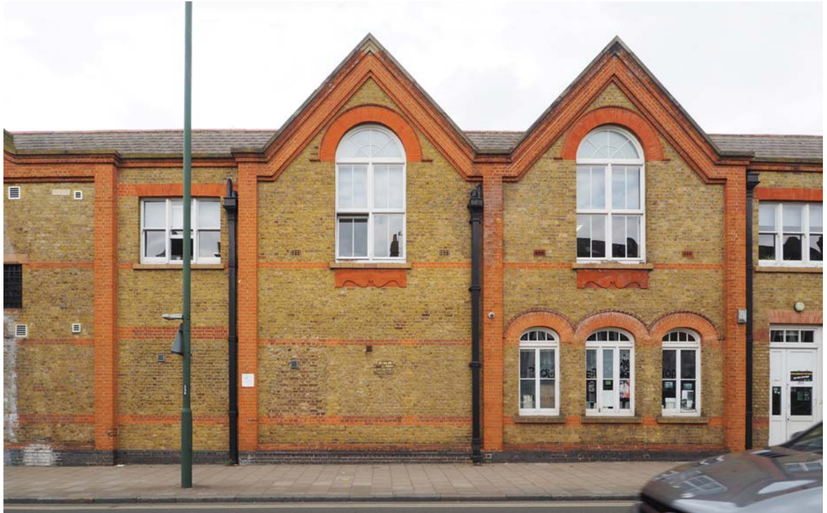
Left to right image 2, South Elevation of The Old Power Station
