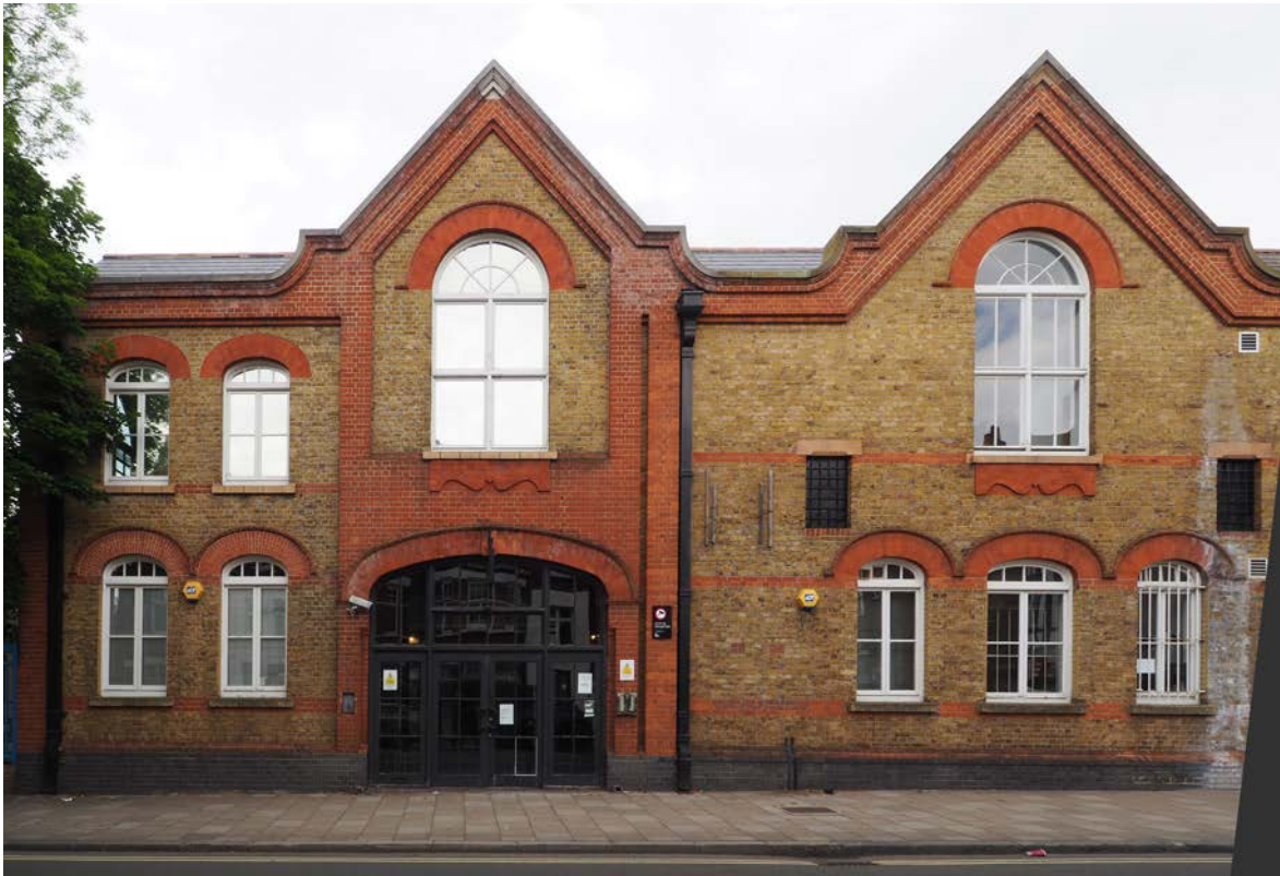
Left to right image 1, South Elevation of The Old Power Station
