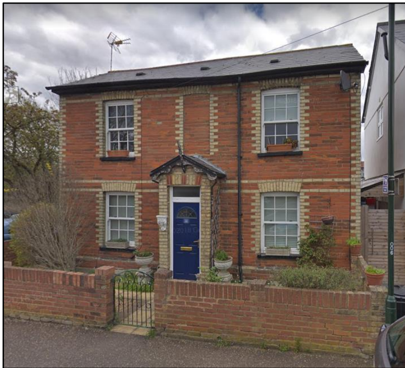
Figure 1 – Front elevation of property.
