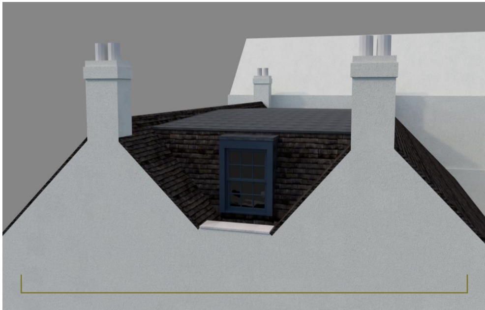
CGI visualisation of proposed scheme showing the modest dormer window to match existing
