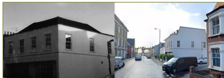
40 Station Road before & after loft conversion
