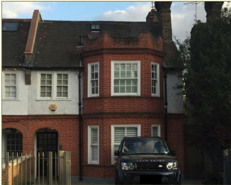
Front elevation of 26 Church Road before conversion
