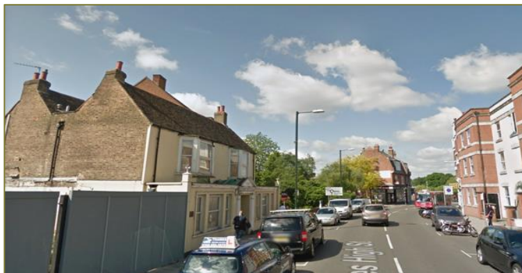
East elevation of No.29 Barnes High Street, infilled by the above scheme in 2017
