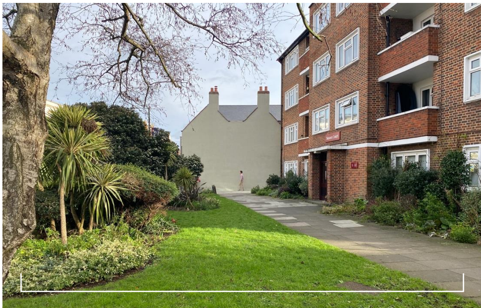
Side elevation of No. 29 Barnes High Street. Roof of No. 28 shown filling the gap between the gable ends
