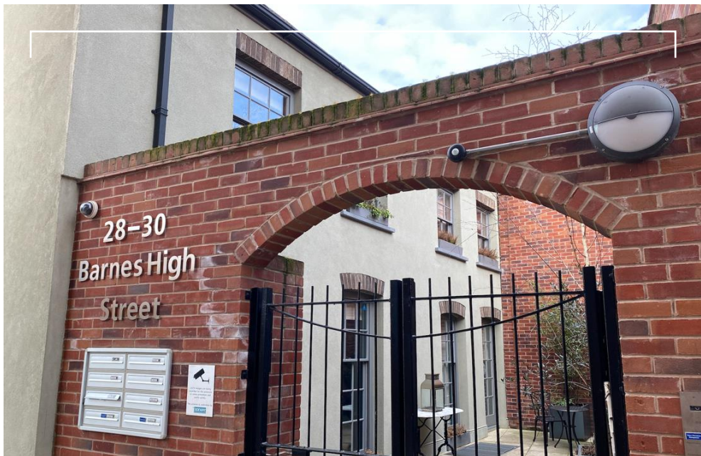
Rear elevation of No. 29 Barnes High Street showing communal courtyard
