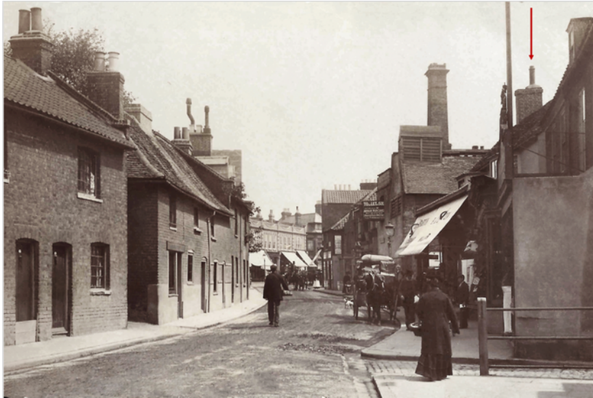
Late C19 photograph showing no.29 with its Victorian shopfront flanked by taller buildings either side.
