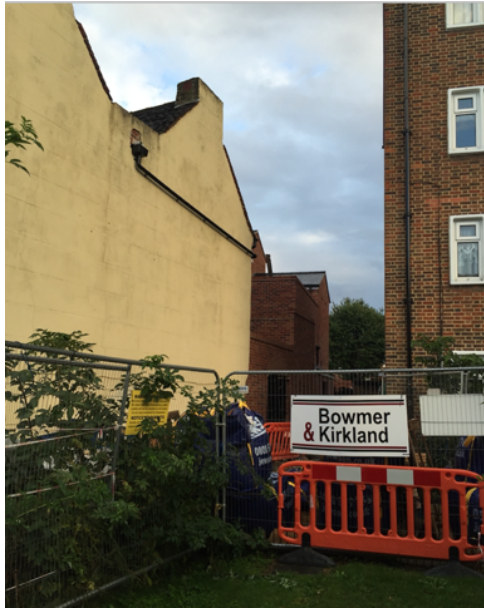
The East side elevation prior to enhancements
