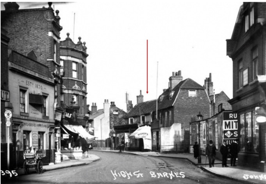
Early C20 photograph showing the 3 storey house (with a half hipped roof and a sash window in the gable end) that once stood immediately to the east of no. 29.
