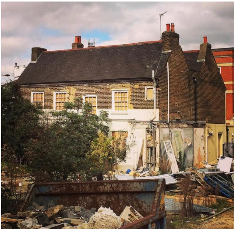
View of rear elevation in 2016, prior to applicants' enhancements.
