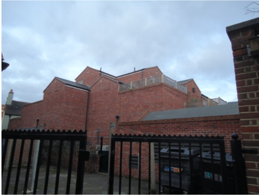
View of rear of the recent development behind the Site – the rear roof of no. 29 can be seen to the far left (facing)
