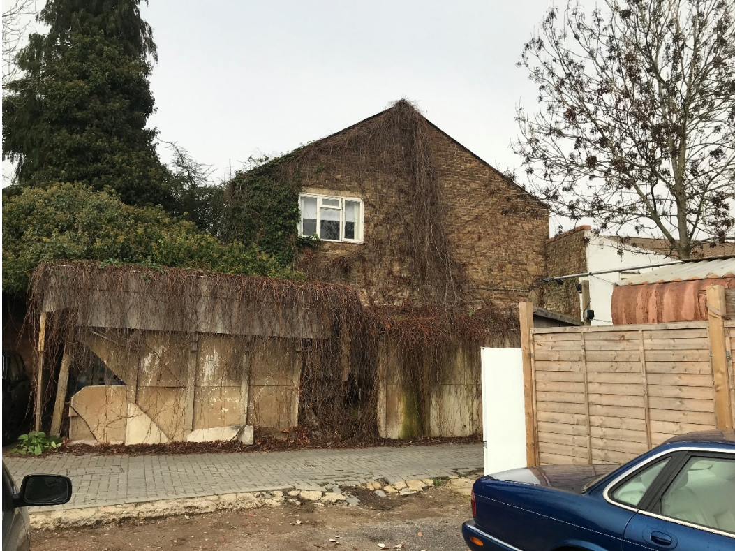
Figure 11: Unsightly dilapidated buildings on the application site (looking north)
