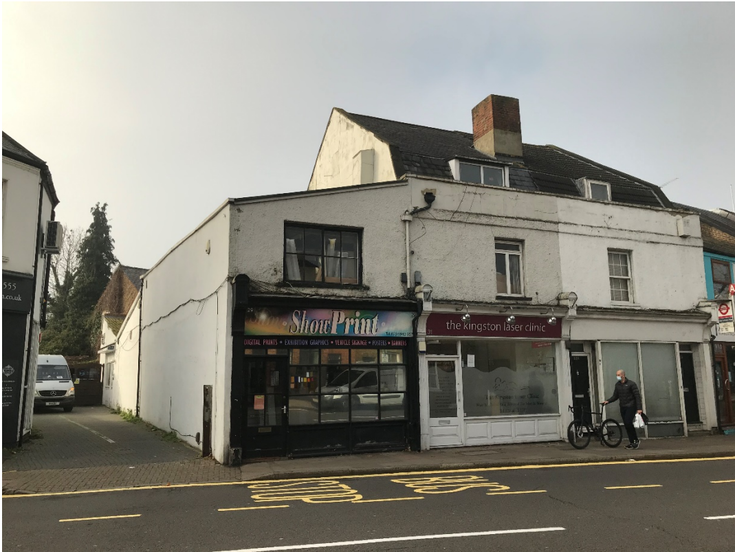
Figure 4: Application Site Buildings with side passage to rear of site
