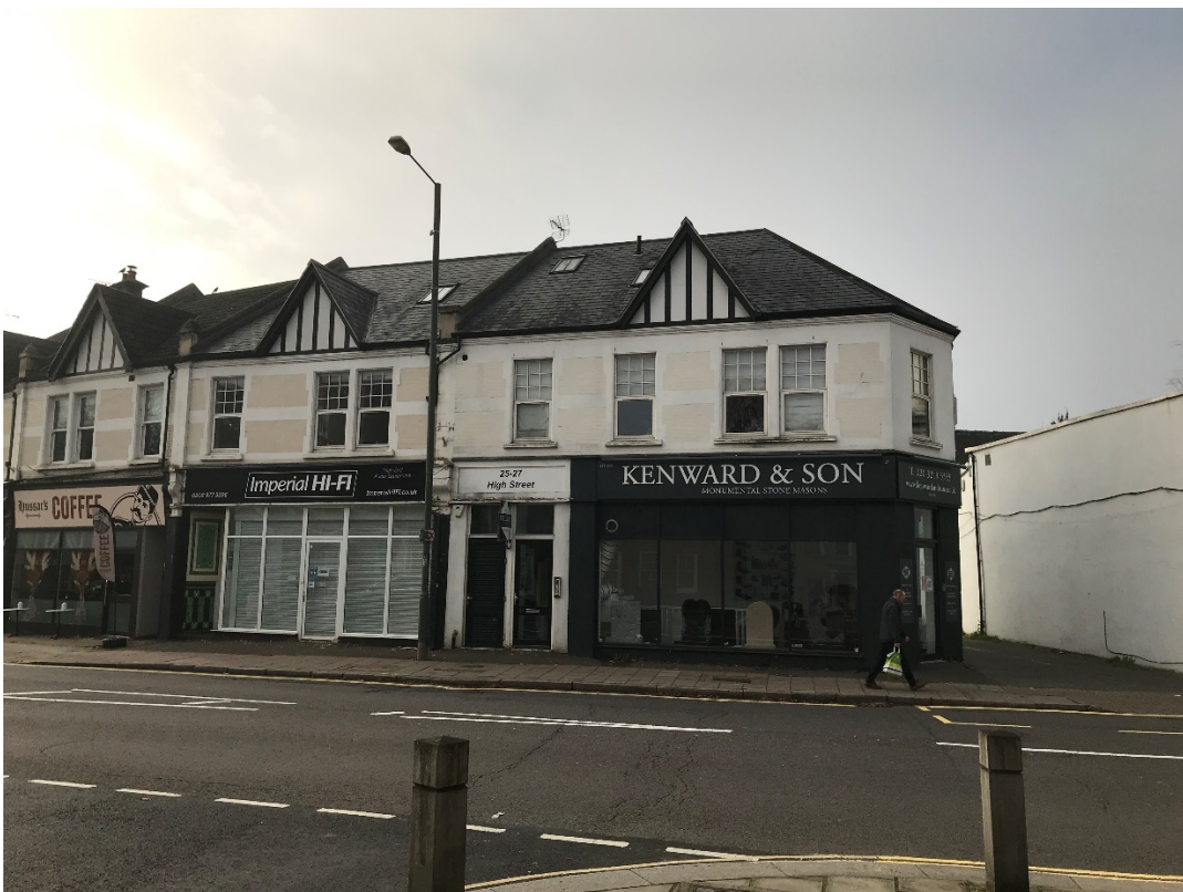
Figure 5: Nos.23-27 High Street, south of application site
