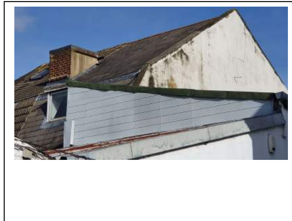
11. Roof to 31, rear elevation
