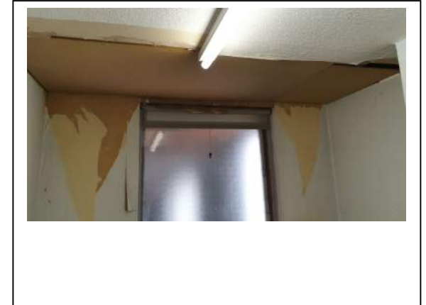
60. Repaired soffit 1 st floor rear room no 31
