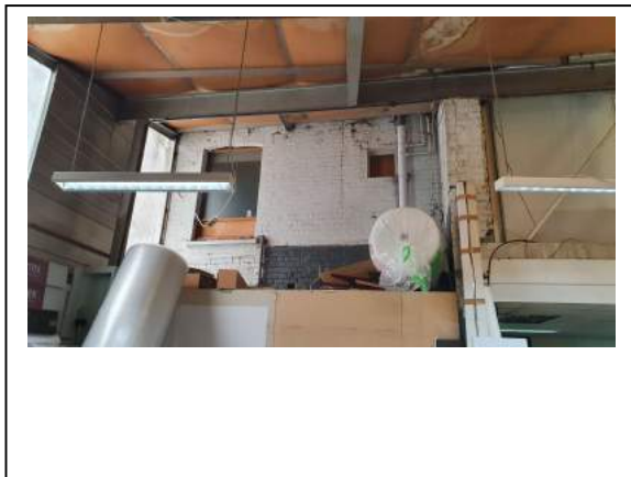
40. Rear elevation of 31 overlooking ground rear of 29
