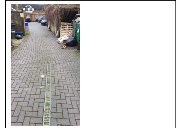
36. Hardstanding with aco slot drain
