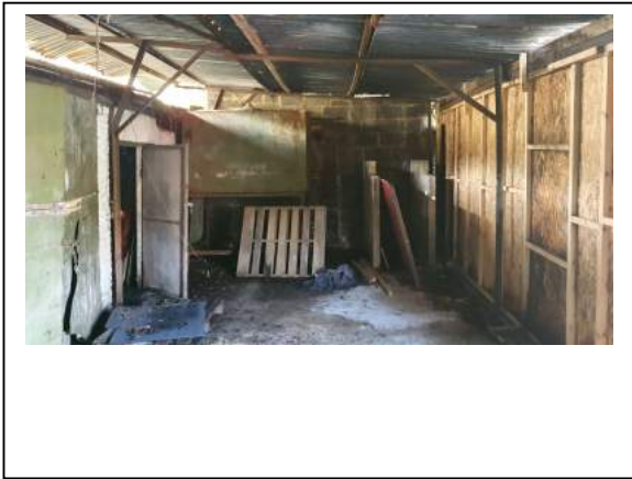
31. Chipboard elevation & doors
