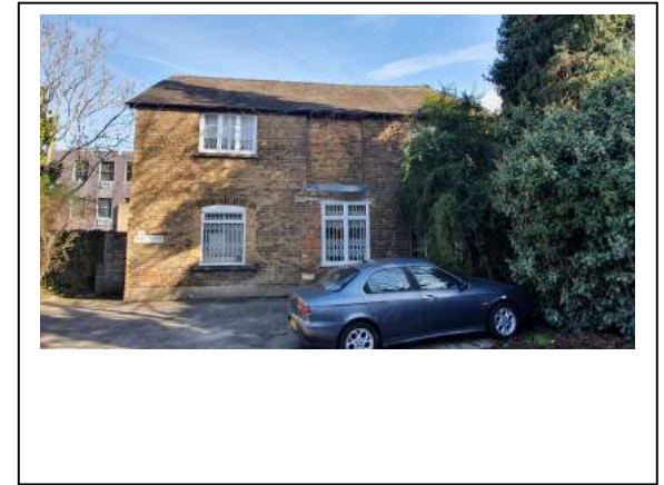
9. North elevation of 29B
