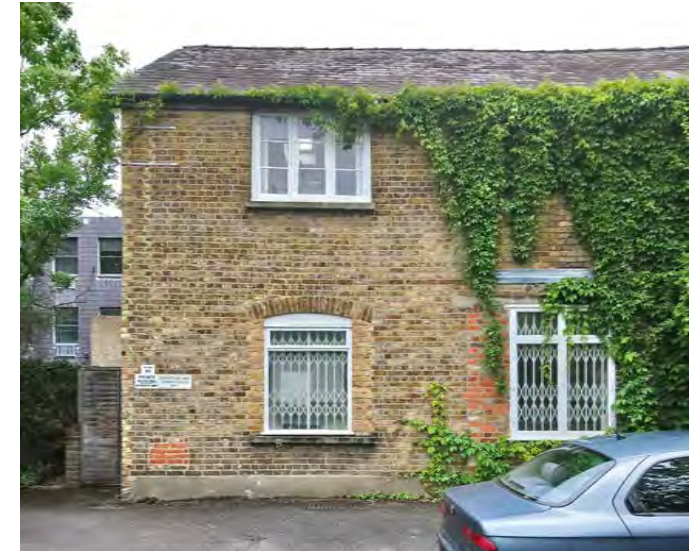
5 - Office building on site
