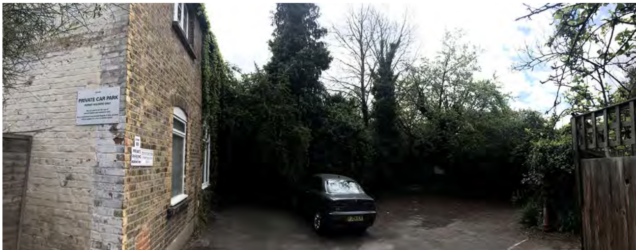
6 - Office building and western boundary
