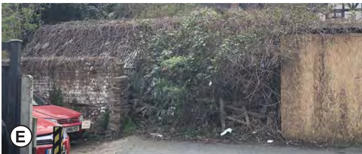
Dilapidated and overgrown structures on site
