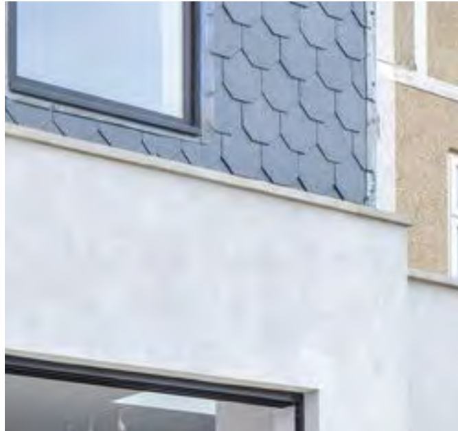
Wall hung slate tiles & Render finish
