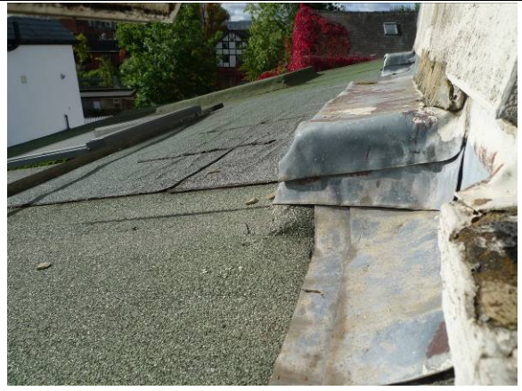
Photo 2 – Flat roof on the eastern elevation of Building B1.
