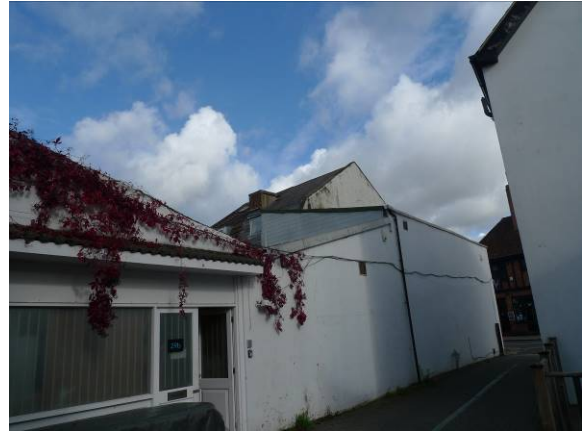
Photo 8 – Building B1 in the background with Building B1 and B2 attached at second storey level.
