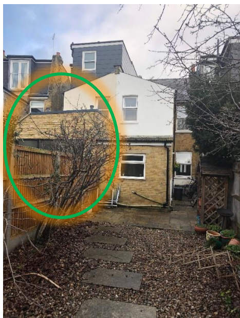
Ground floor Rear extension as built at property No. 7 Bushy Park Road (End of terrace property)
